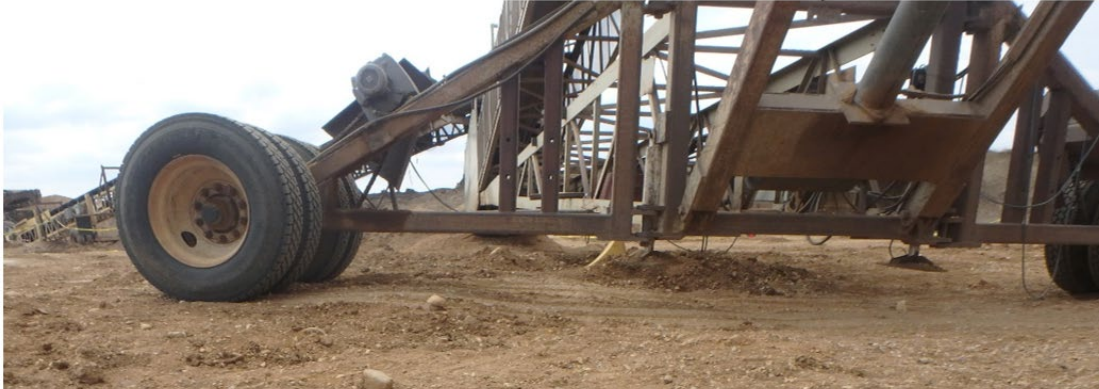
Radial stacker at east end of travel in runway.
