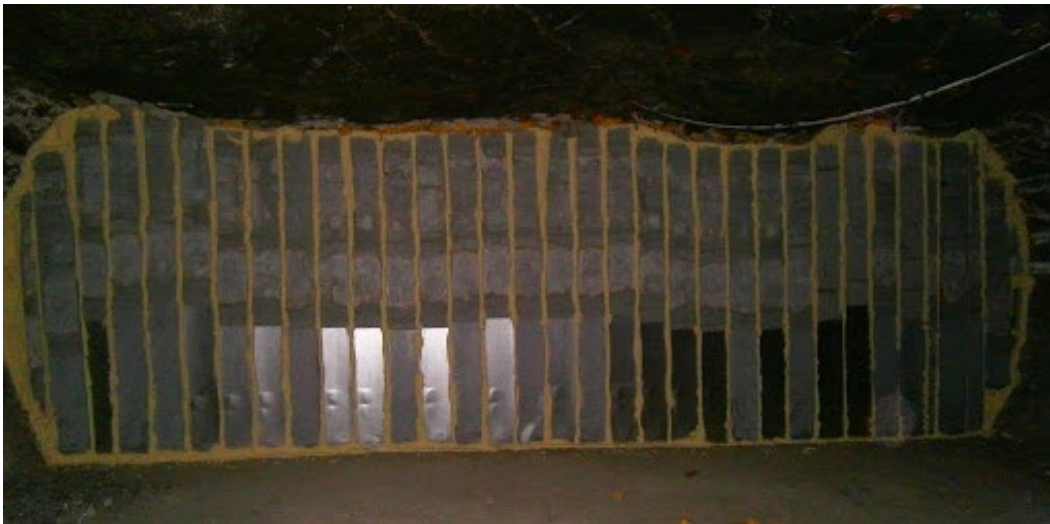
Visual 8-3 - Stopping with Sealant
