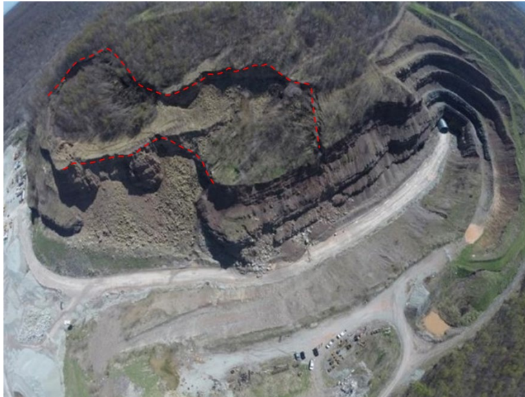
Figure 2. Aerial view of Mine A subsidence
