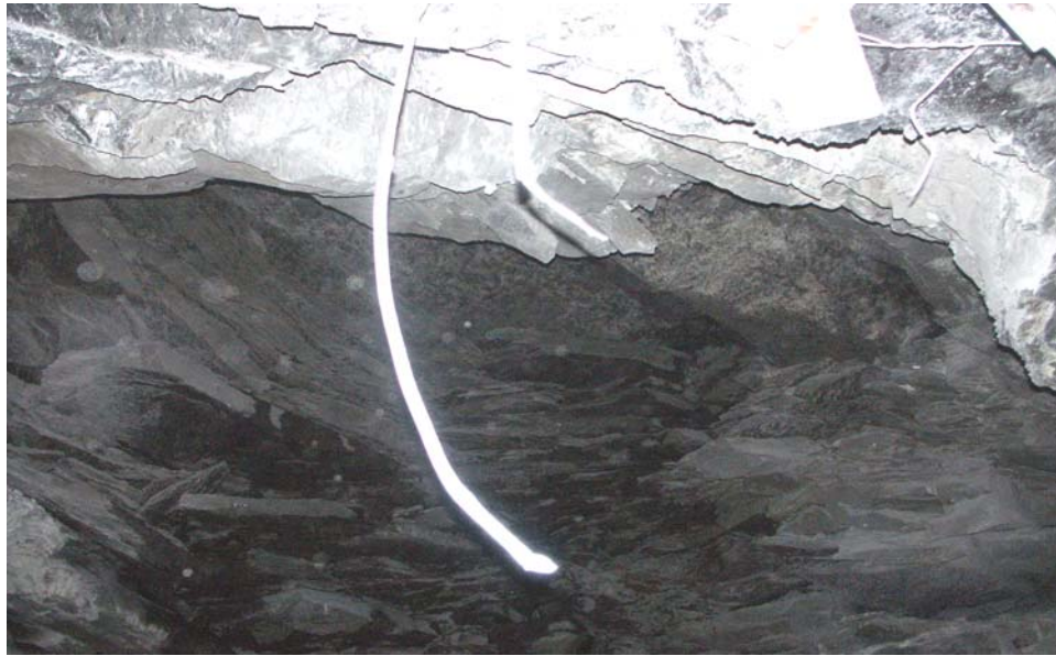
View of rock fall in No. 2 Entry of 4 Section showing broken cable roof bolt.
