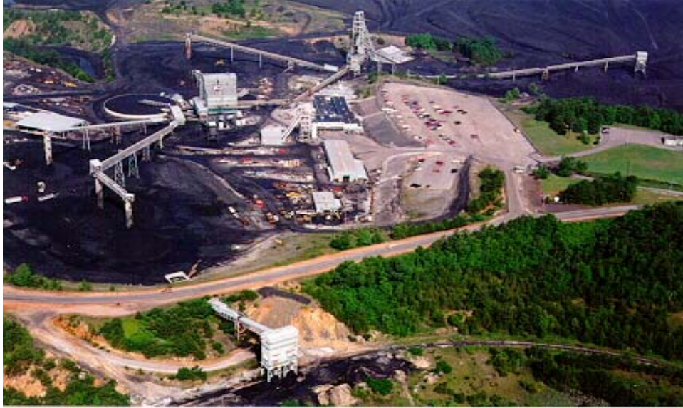
Jim Walter Resources, Inc., No. 5 Mine aerial view.
