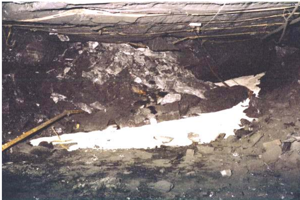
No. 2 Entry showing inby side of rock fall in 4 Section.
