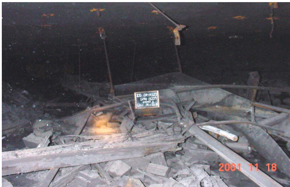
No. 3 Entry showing destructive forces looking out by in 4 Section.
