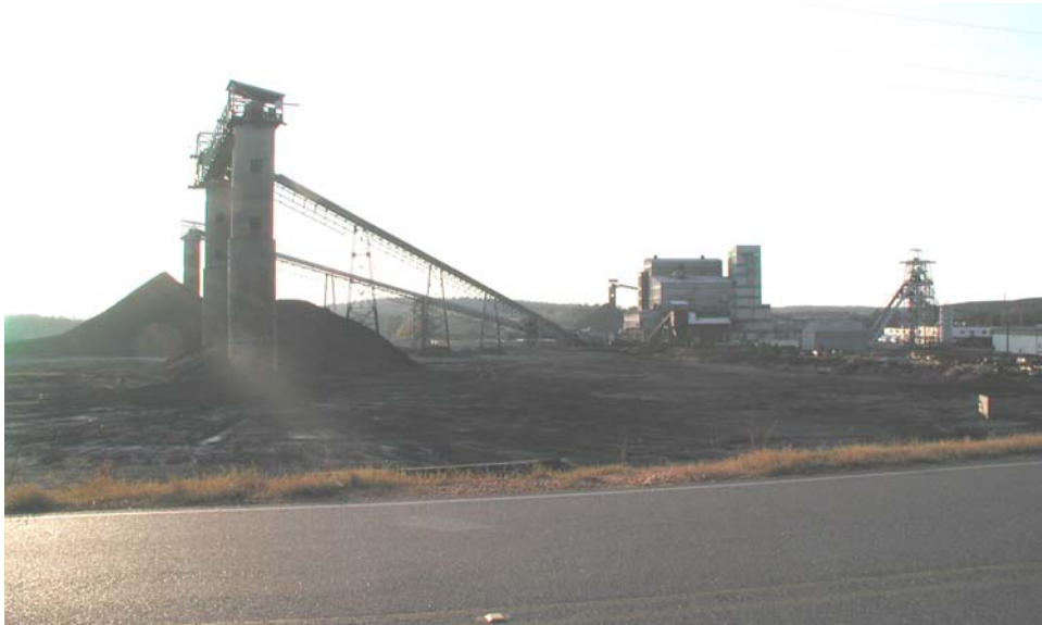
Jim Walter Resources, Inc., No. 5 Mine ground view.
