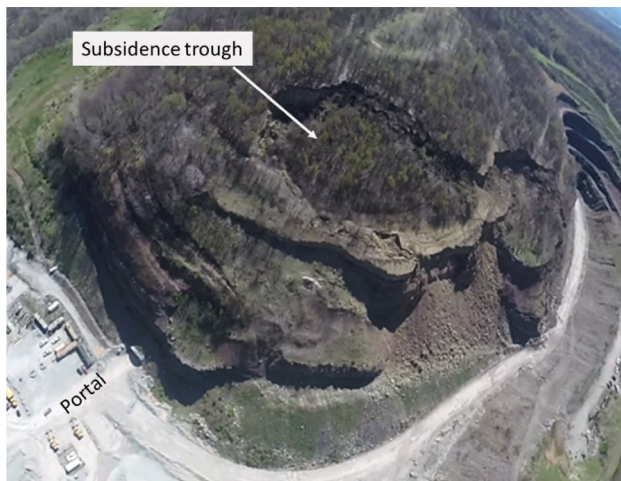
Fig. 1 Aerial view of the mine showing extent of surface subsidence associated with the collapse of the pillars
