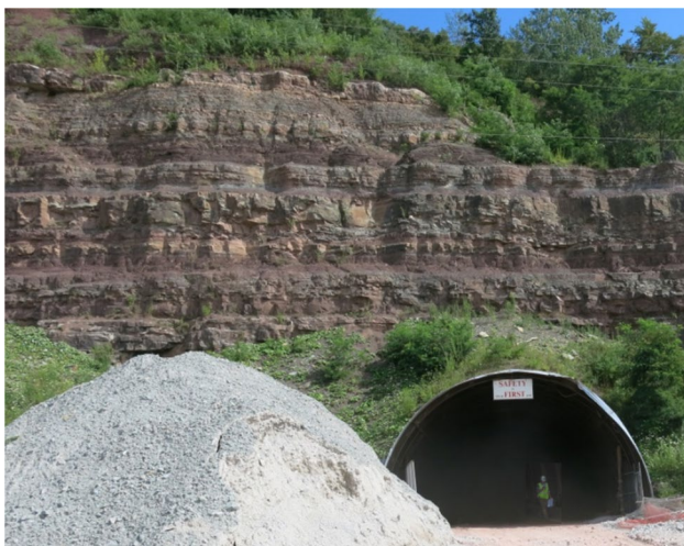
Fig. 3 Access portal entering the mine with Mauch Chunk beds exposed in the highwall
