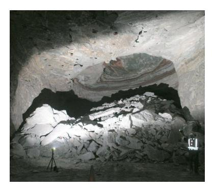
**Figure 32.** Large stress-related, oval-shaped fall that has propagated upwards into weaker, overlying strata in a limestone mine.
