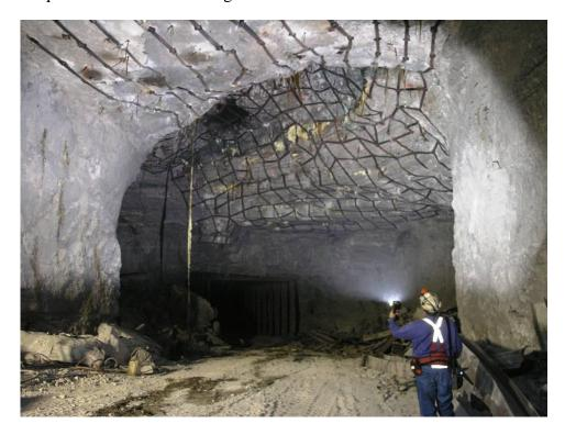
**Figure 28.** Bolts, straps, and injection grouting used to rehabilitate the roof at the site of a major roof fall.
