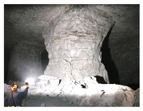
**Figure 3.** Partially benched pillar failing under elevated stresses at the edge of bench mining. Typical hourglass formation indicates overloaded pillar. The width-to-height ratio is 0.44 based on full benching height and the average pillar stress is about 12% of the UCS.
