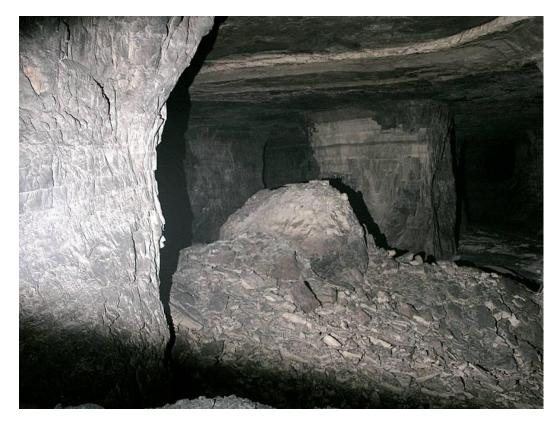
**Figure 6.** Remaining stump of a collapsed pillar in an abandoned area. Thin, weak beds in the pillar and moist conditions are thought to have contributed to the failure. The width-to-height ratio was 0.82 and average pillar stress about 11% of the UCS.
