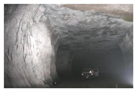
**Figure 7.** Example of rib spalling and resulting concave pillar ribs that can initiate when average pillar stress exceeds about 11% of the UCS.
