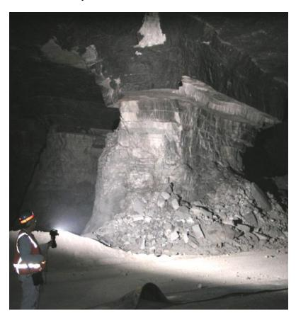
**Figure 17.** Pillar damage observed in rock containing thin, weak bands. Note spalling of the intact rock material between the weak bands.
