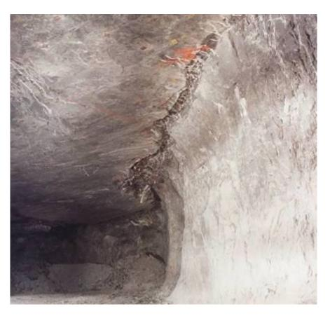
**Figure 31.** Roof guttering at the pillar-roof contact.
