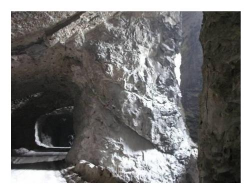
Figure 13. Example of a pillar that is bisected by a large, angular discontinuity.
