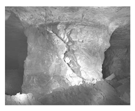
**Figure 4.** Partially benched pillar that failed along two angular discontinuities. Width-to-height ratio is 0.58 based on full benching height; average pillar stress is about 4% of the UCS.
