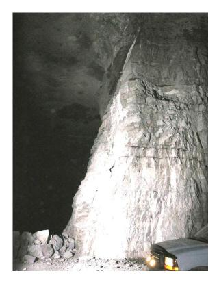
**Figure 15.** Loss of pillar rib at the location of a large roof-to-floor discontinuity in a limestone mine.
