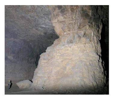
**Figure 14.** Rib failure related to large, angular discontinuities adjacent to a fault zone.
