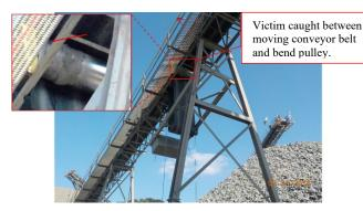
A miner suffered fatal injuries in 2018 when he was entangled in a conveyor's take-up assembly. He was working from an elevated aerial lift cleaning buildup from a bend pulley while it was operating.
