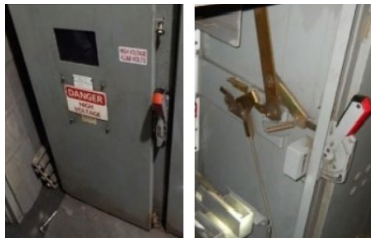
Linkage adjusted with circuit energized.
