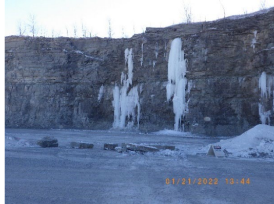
A miner was severely injured while working near the base of an approximate 65 ft. highwall. The miner was struck by loose, fractured and overhanging rocks.
