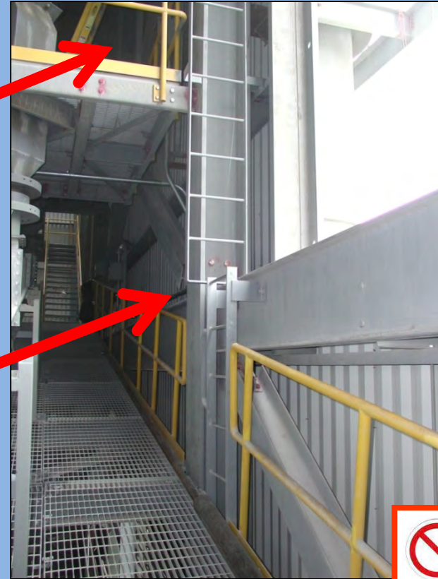
Ladder access and divided ladder sections
