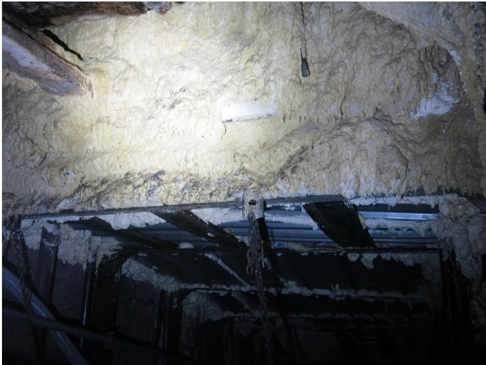
Foam injected into a cavity above steel sets.
