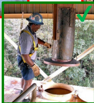
Far right: Safe - Dual lanyards used for tie-off when working and moving at height
