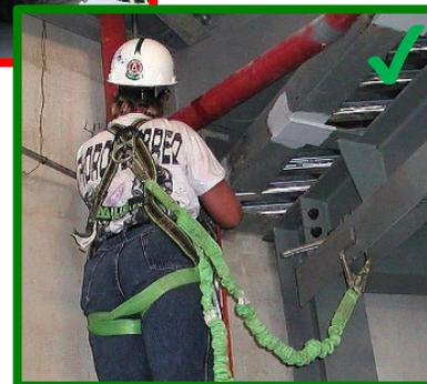
*Far right: Safe - Dual lanyards used for tie-off when working and moving at height*
