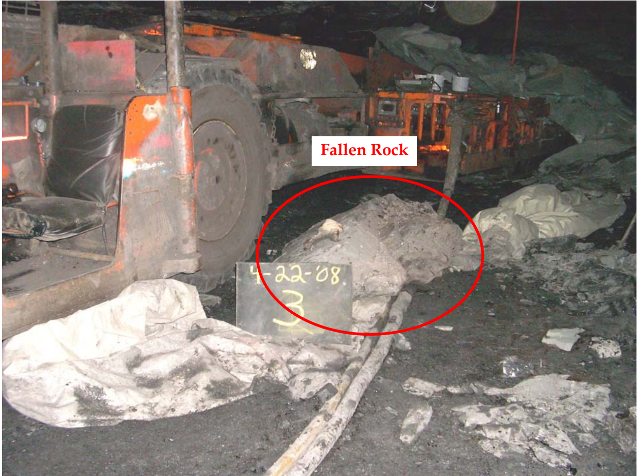
Photograph 1 - Fallen Roof and Rib Rock
