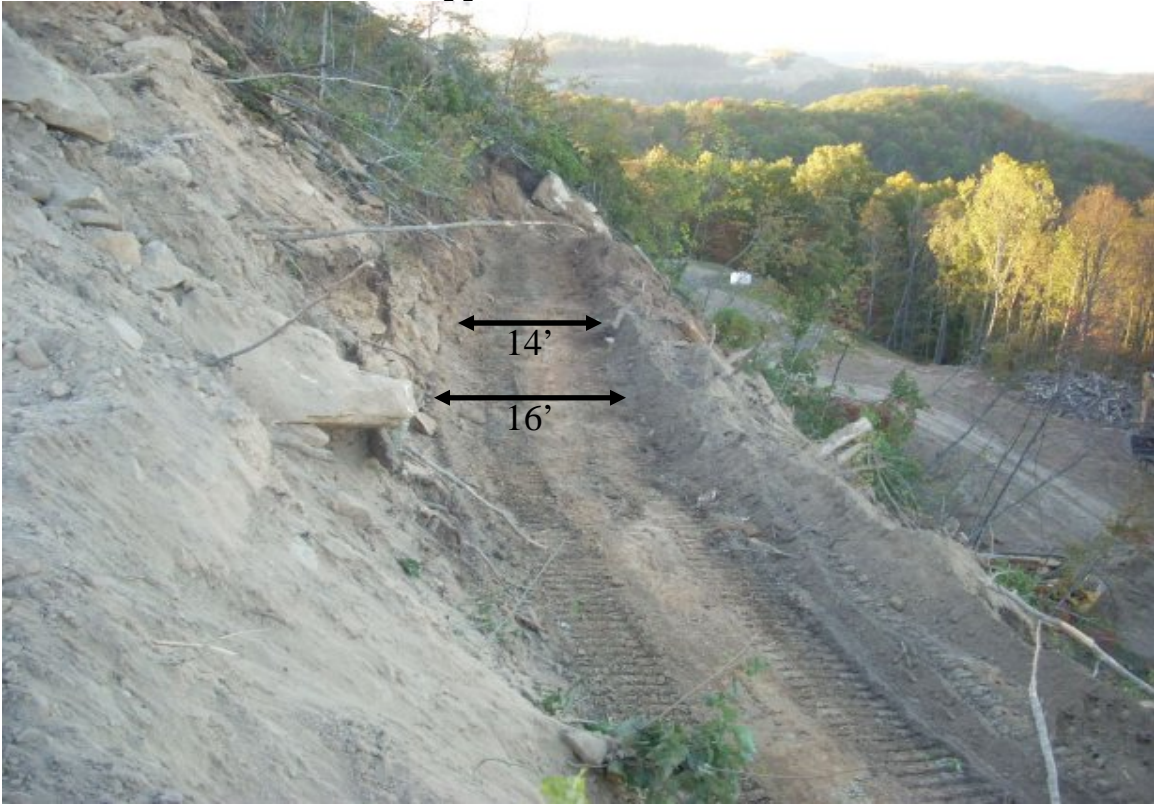
BENCH UNDER CONSTRUCTION
