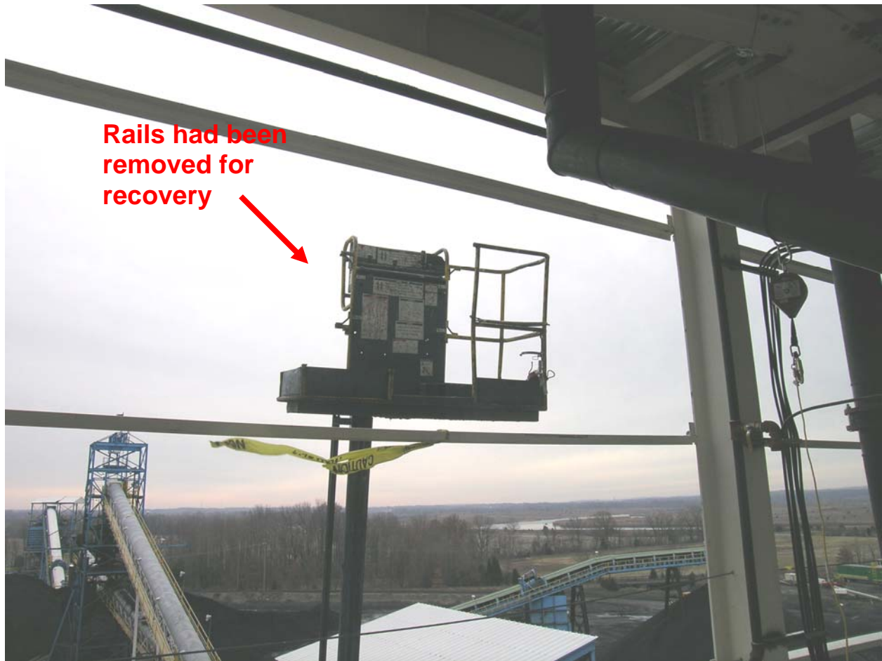
View from inside of the plant approximate post accident position of platform.
