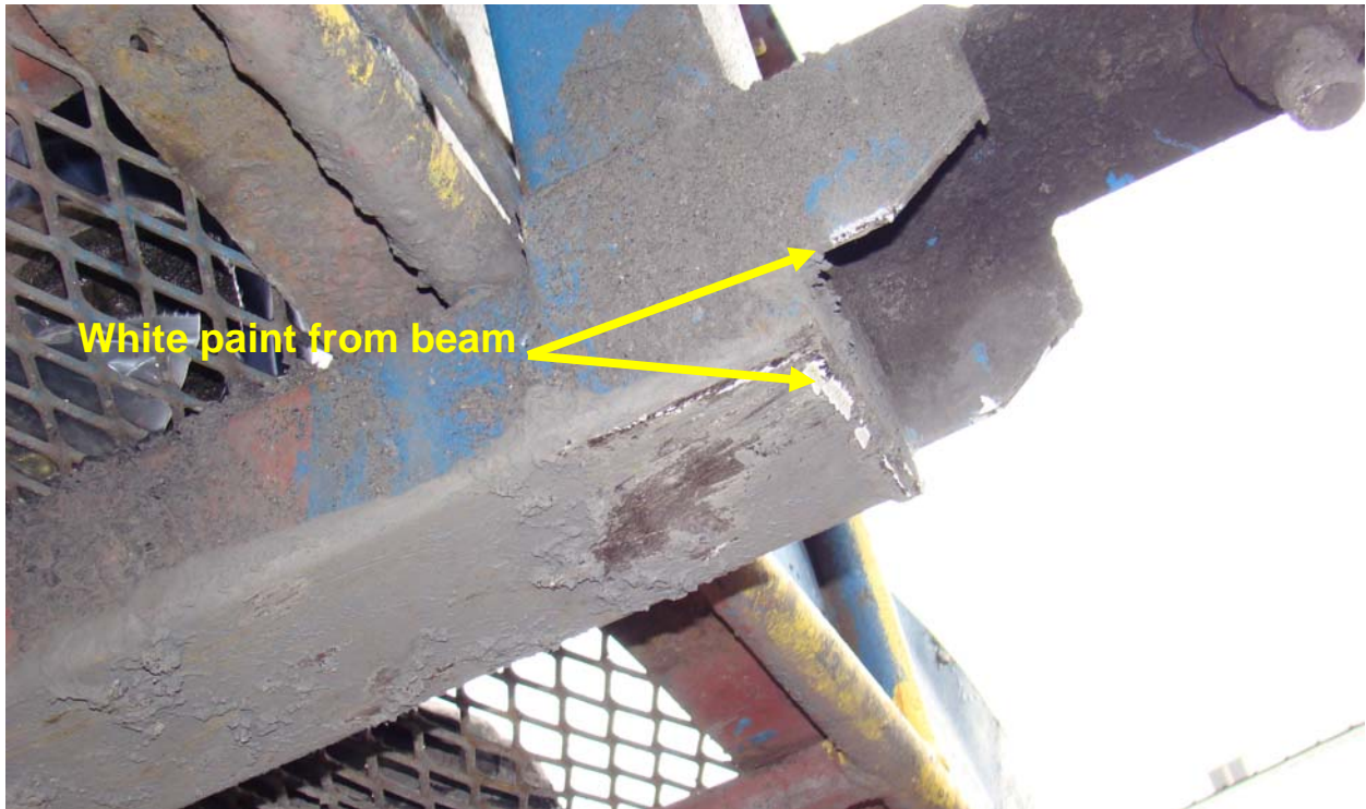
Photograph depicts white paint from the beam on the knuckle of the platform
