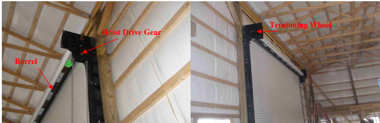
Figure 2. Door views – drive gear side (l), tensioning wheel side (r).
