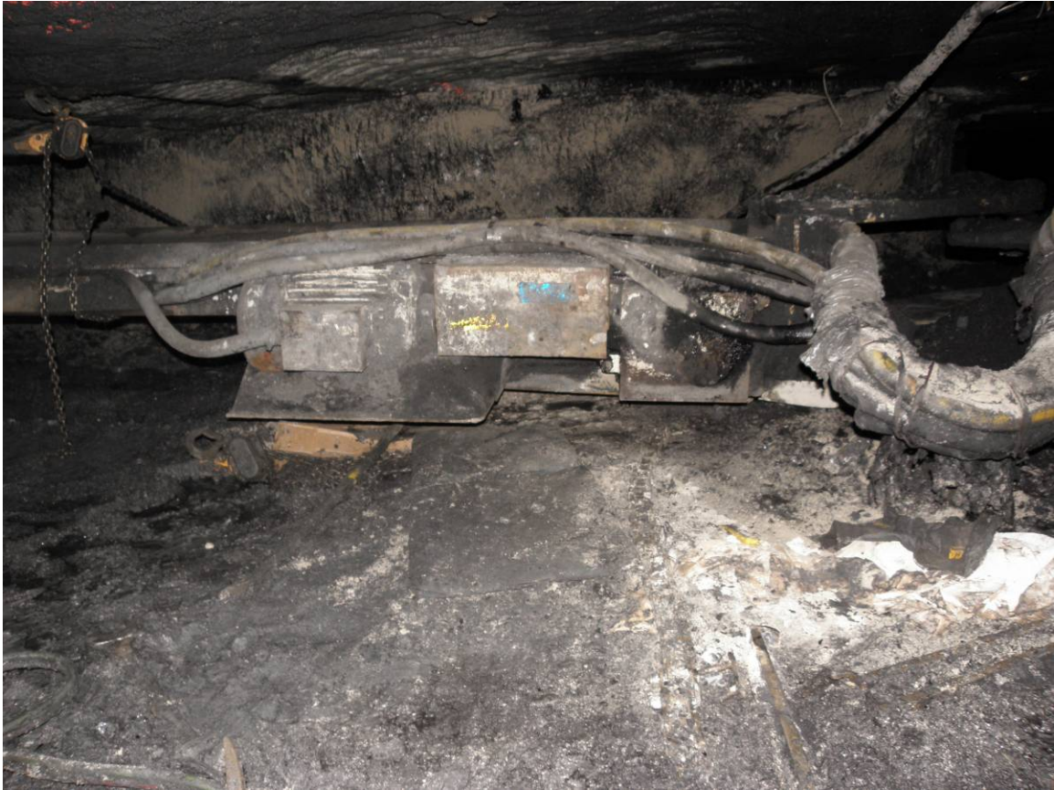
Photo of Accident Site
