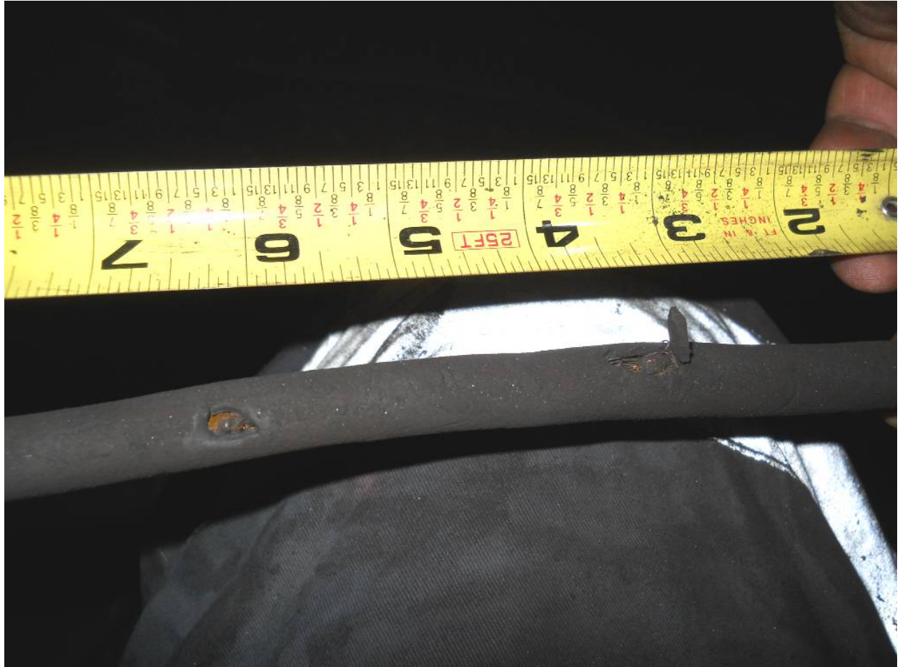
Photo 2 - Damaged Welding Lead
