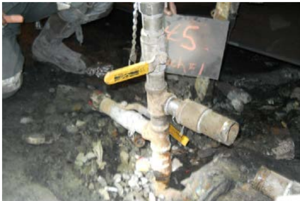
Water manifold reinstated during investigation
