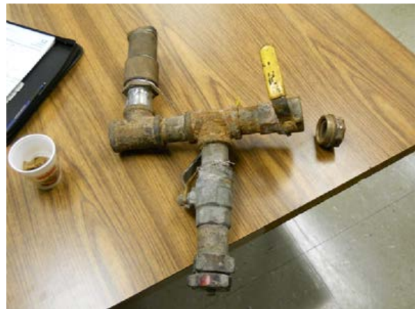
Photo depicts the actual valve separation
