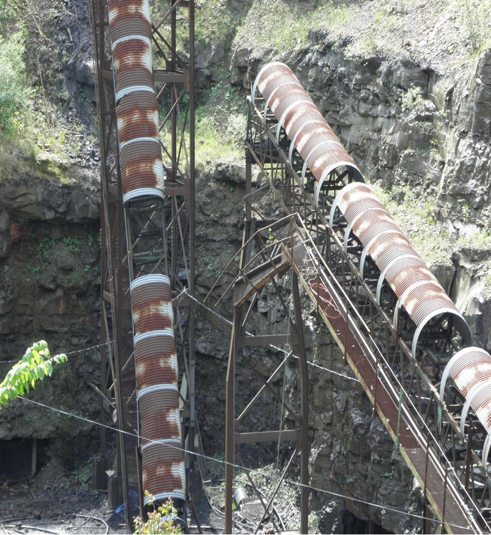
Photograph of accident scene
