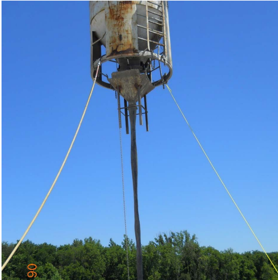
Photograph showing the concrete bucket, hopper, and 8" flexible hose
