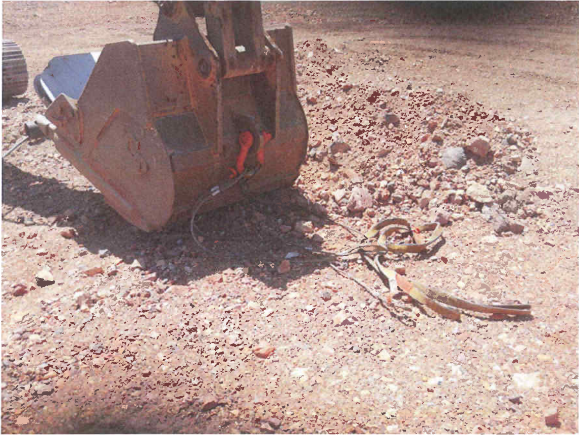
Photograph 4: Straps and Excavator Used To Make a Basket to Remove Rock
