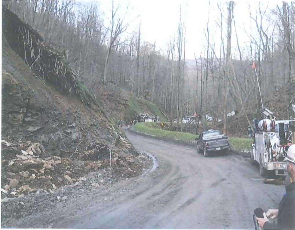
View of the accident scene looking down the Eagle Land haul road
