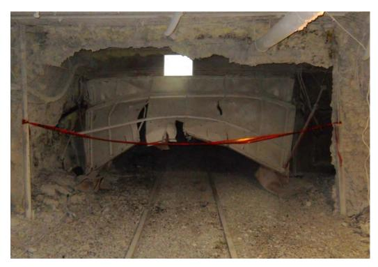
Meddings, the locomotive, and six cars crashed through this outby airlock door. This photograph shows the door from the outby side and is opposite to the direction the train was traveling.
