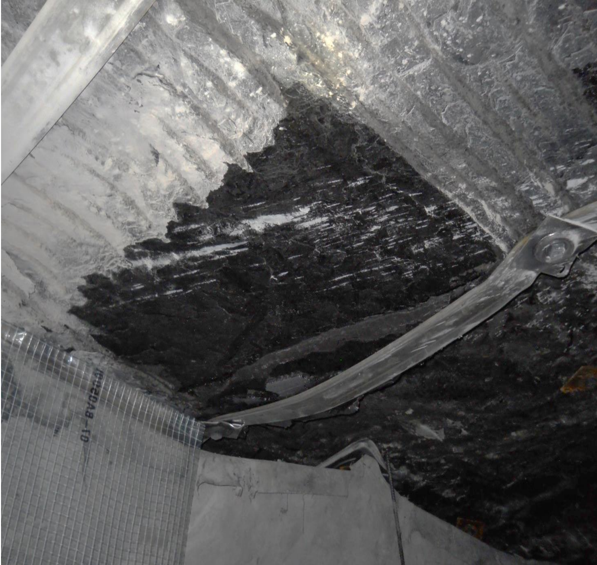
PHOTO OF ROOF AT ACCIDENT SCENE
