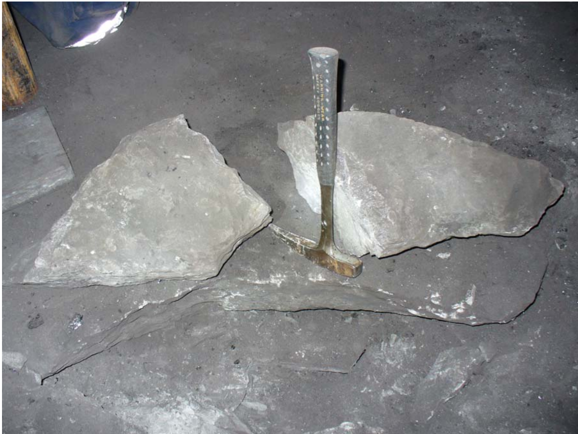
Figure Q-5. Sample of sandstone was collected from floor heave brow beneath survey station 22582 in 1 North Panel longwall tailgate, 36 feet outby the face. Brow of heaved sandstone slab reveals rootless crack.
