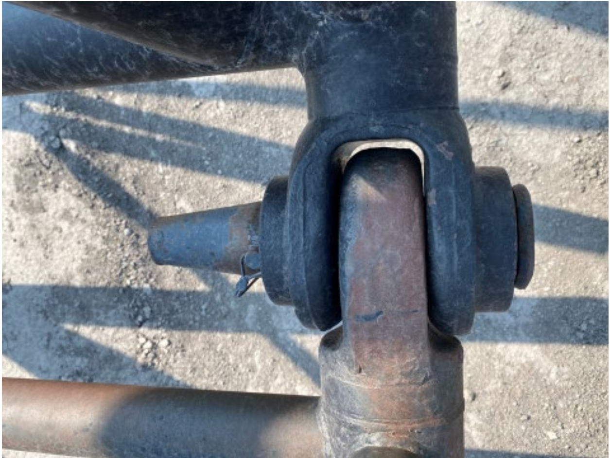
APPENDIX B – Photo of Bottom Left Pin before Removal
