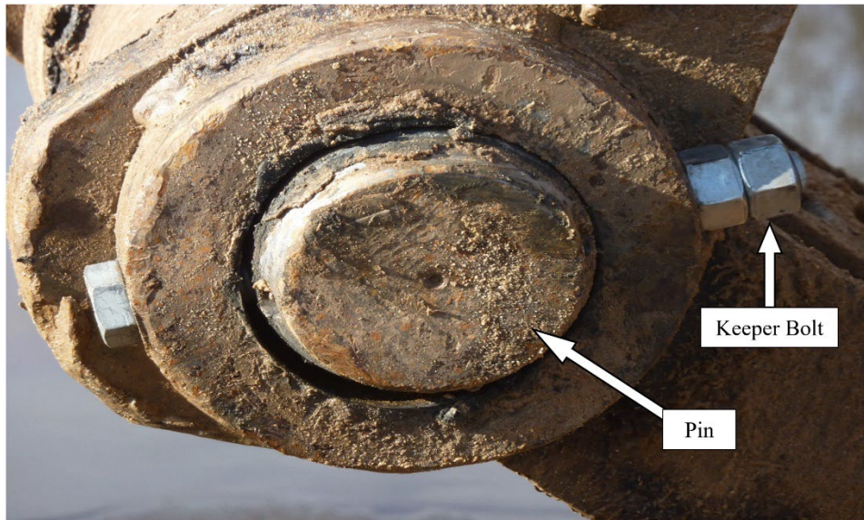
Proper Installation of Keeper Bolt
