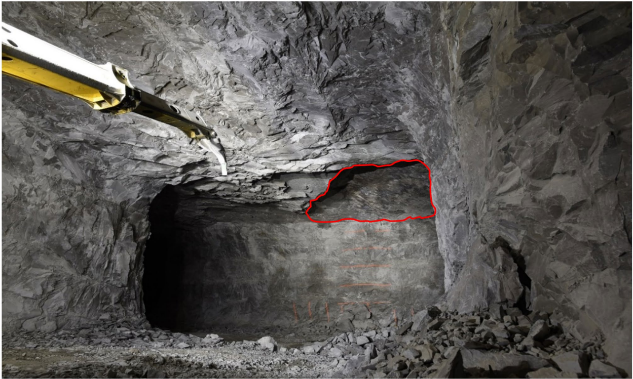
View of rock fall from Crosscut M27 looking Southwest into Heading C19. The red outline indicates the wedge-shaped fall cavity.
