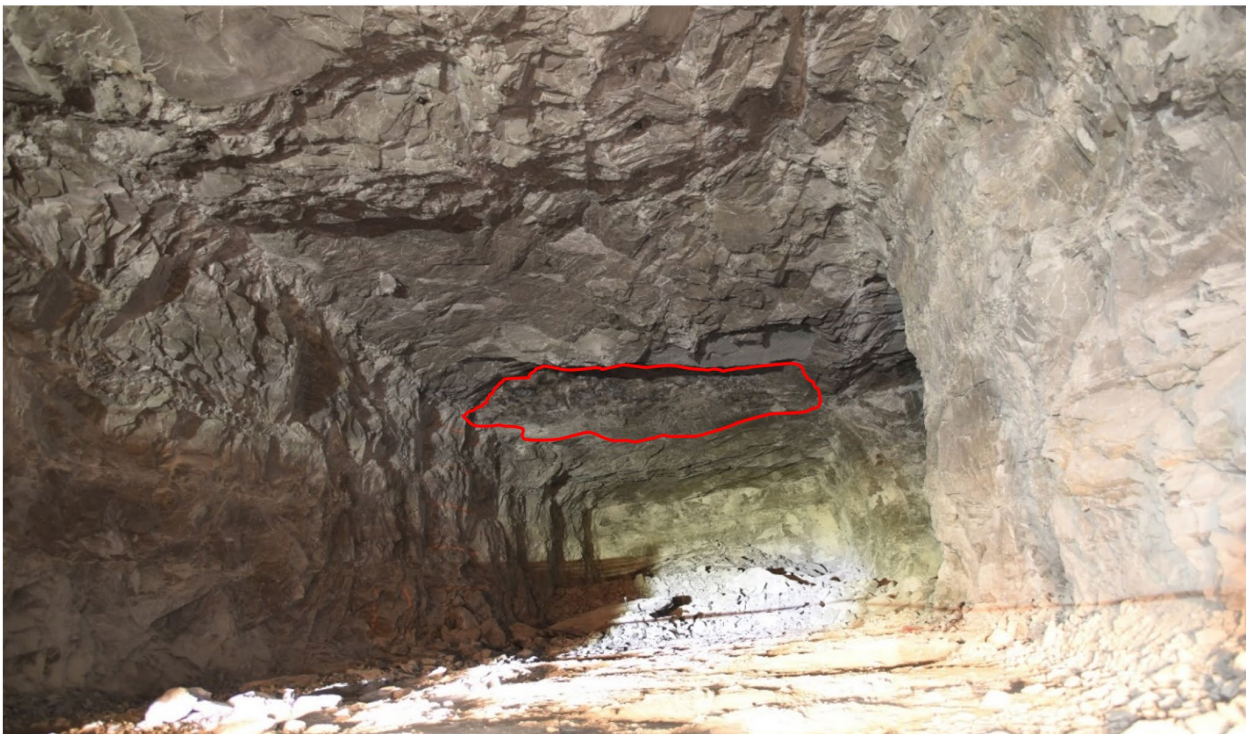
View of rock fall from Heading C19 looking Northwest into face. The red outline indicates the wedge-shaped fall cavity.
