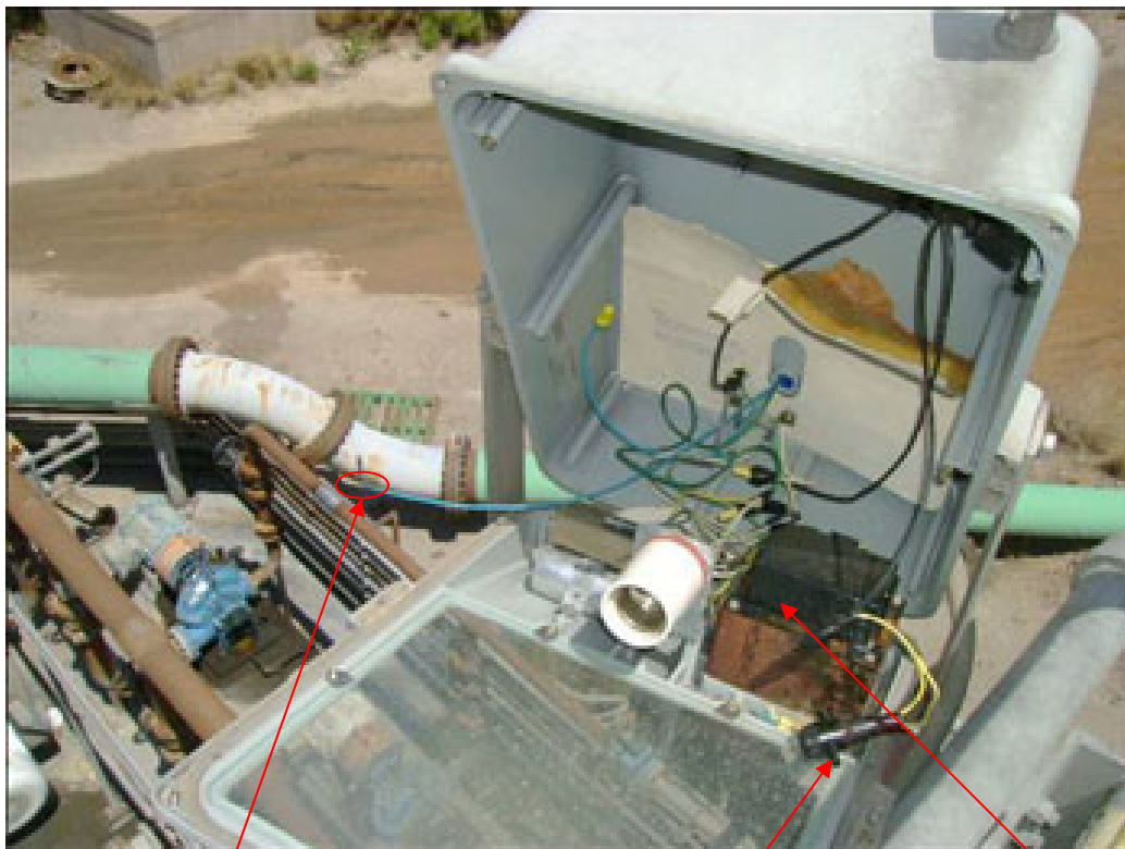
Energized conductor contacted by victim
