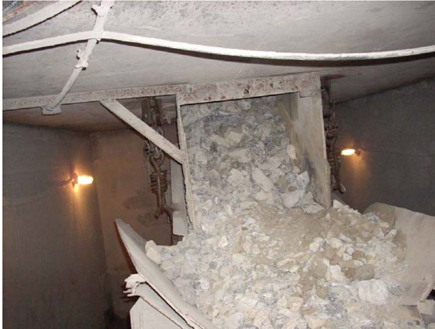
Chute in surge tunnel below primary surge pile
