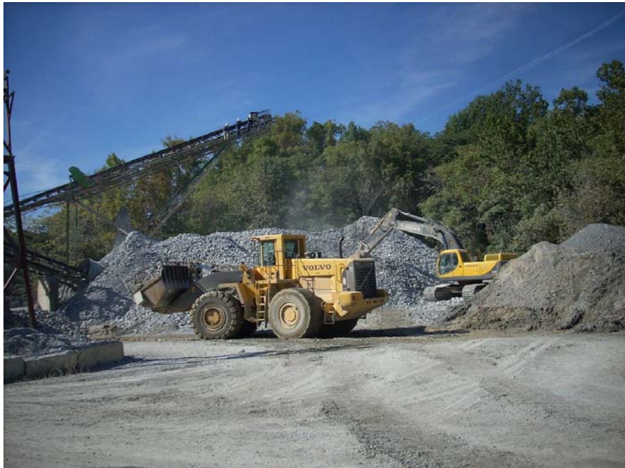
Removal of surge pile over feeder during recovery
