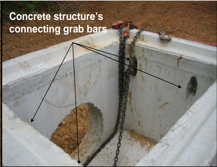
Unrated chain, clevis grab hooks and broken link
