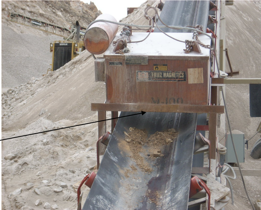
Photograph of Accident Scene
