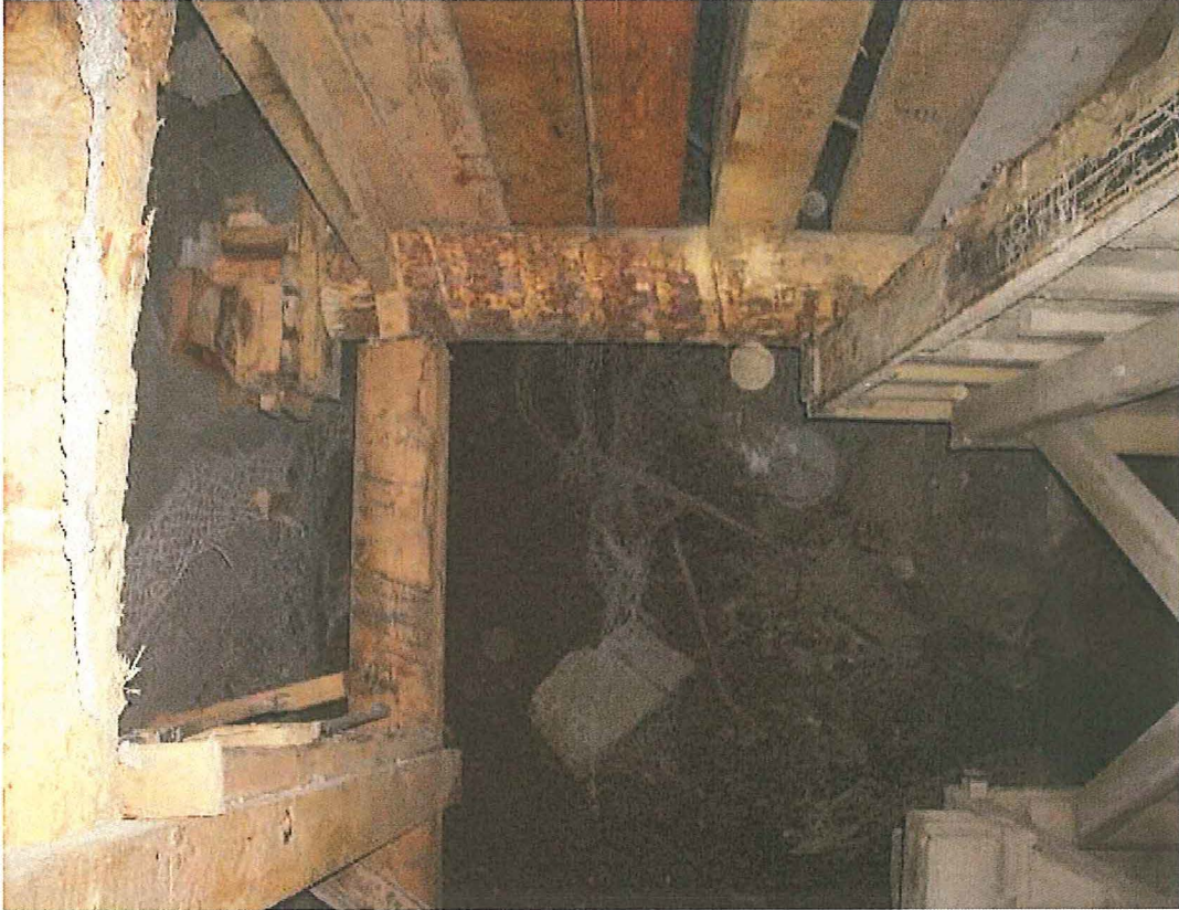
Note: Timbers installed after ground fall.
