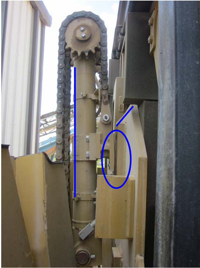
Illustration 3: Bent cylinder, frame plate, and one of the spaces between the counterweight lift mechanism mount and excavator frame.
