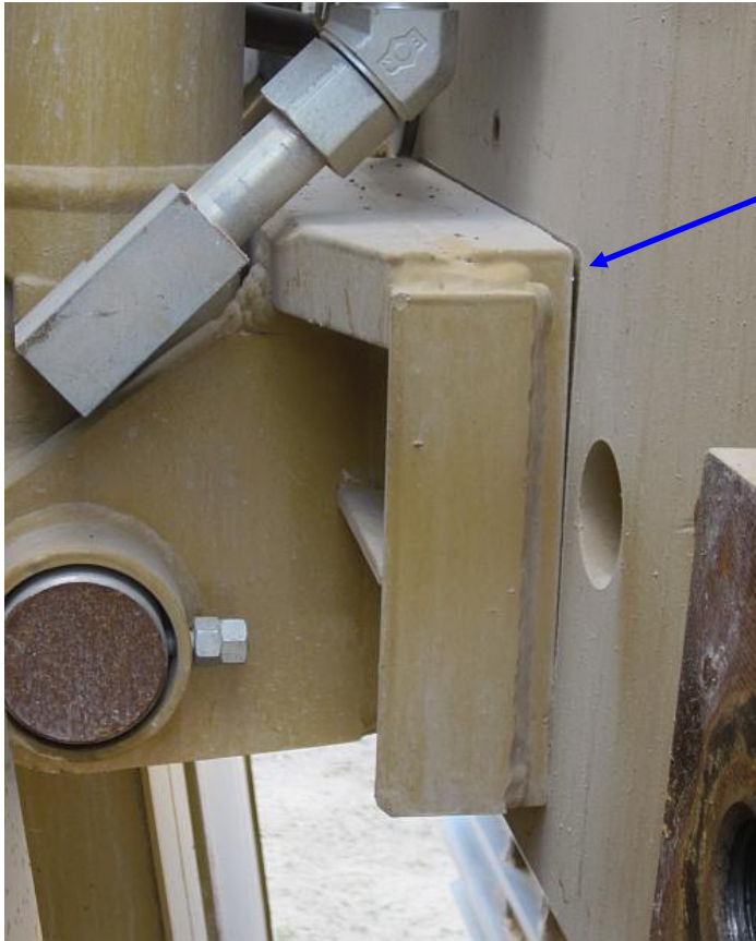
Illustration 4: Close up of one of the spaces between the counterweight lift mechanism mount and excavator frame.
