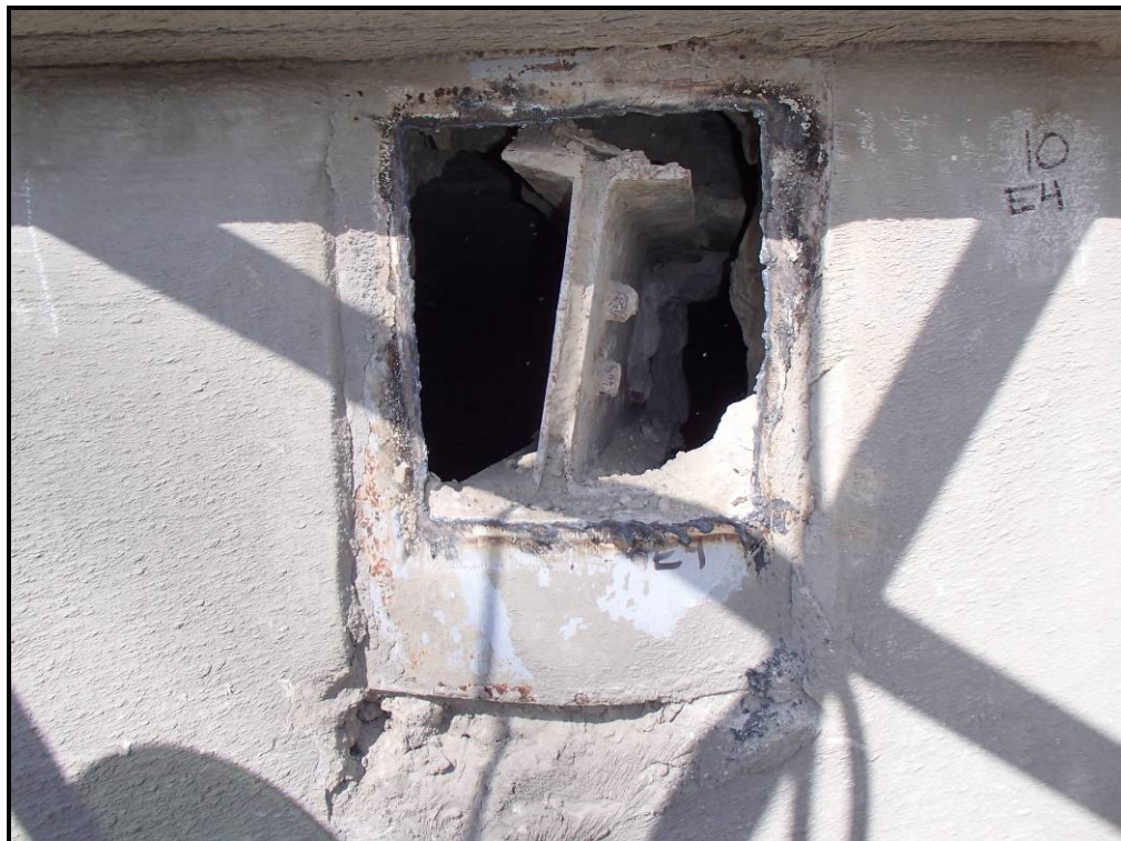
Photo 40 – At East 4 pocket of Silo 10, Beam 4 is rotated and separated from the roof slab by approximately 5 inches.
