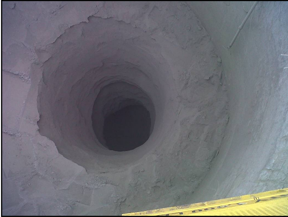
Photo 13 – Stable rathole as Silo 12 was drawn down. Picture taken on September 14, 2012. The flow channel tended toward the east wall.
