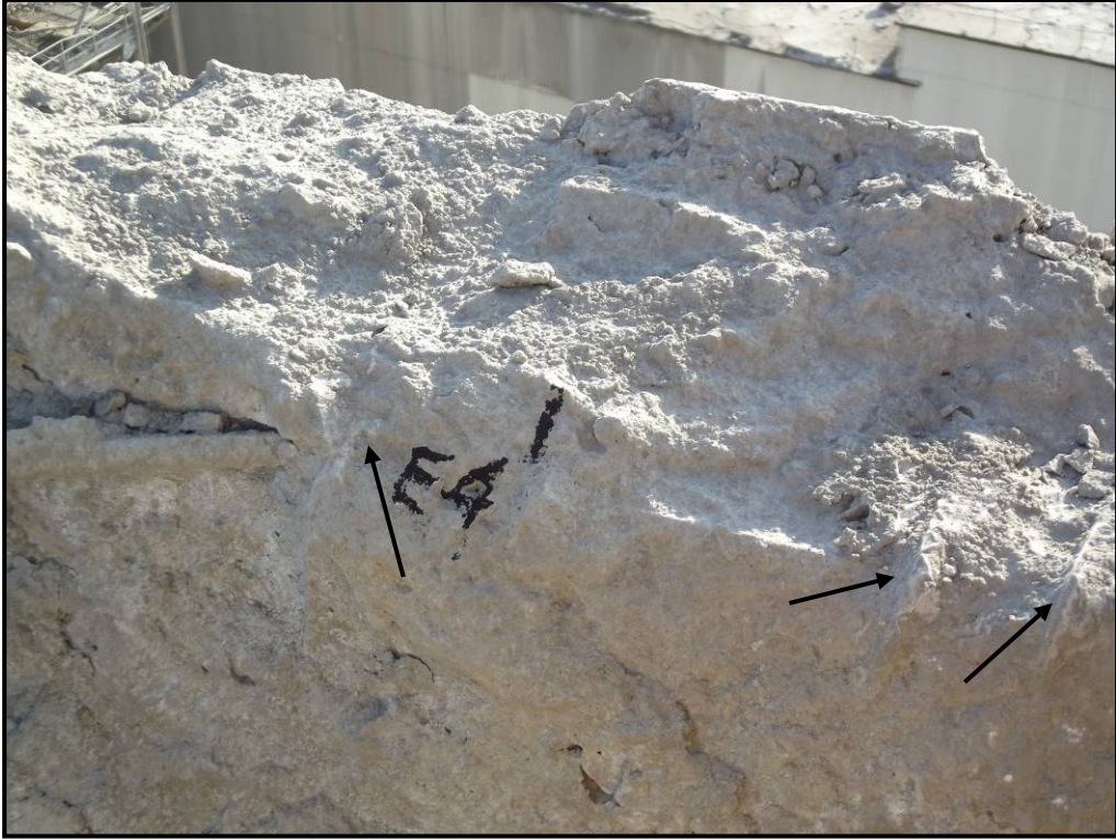
Photo 21 – Silo 12 East 4 pocket completely torn from silo wall above the location of the shear stirrups (arrows)
