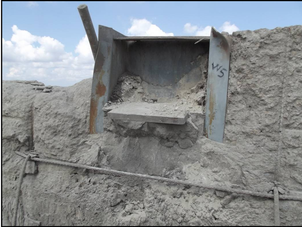
Photo 25 – Silo 12 West 5 pocket bearing plate tilted down and delamination detected in 9 inch layer of grout.
