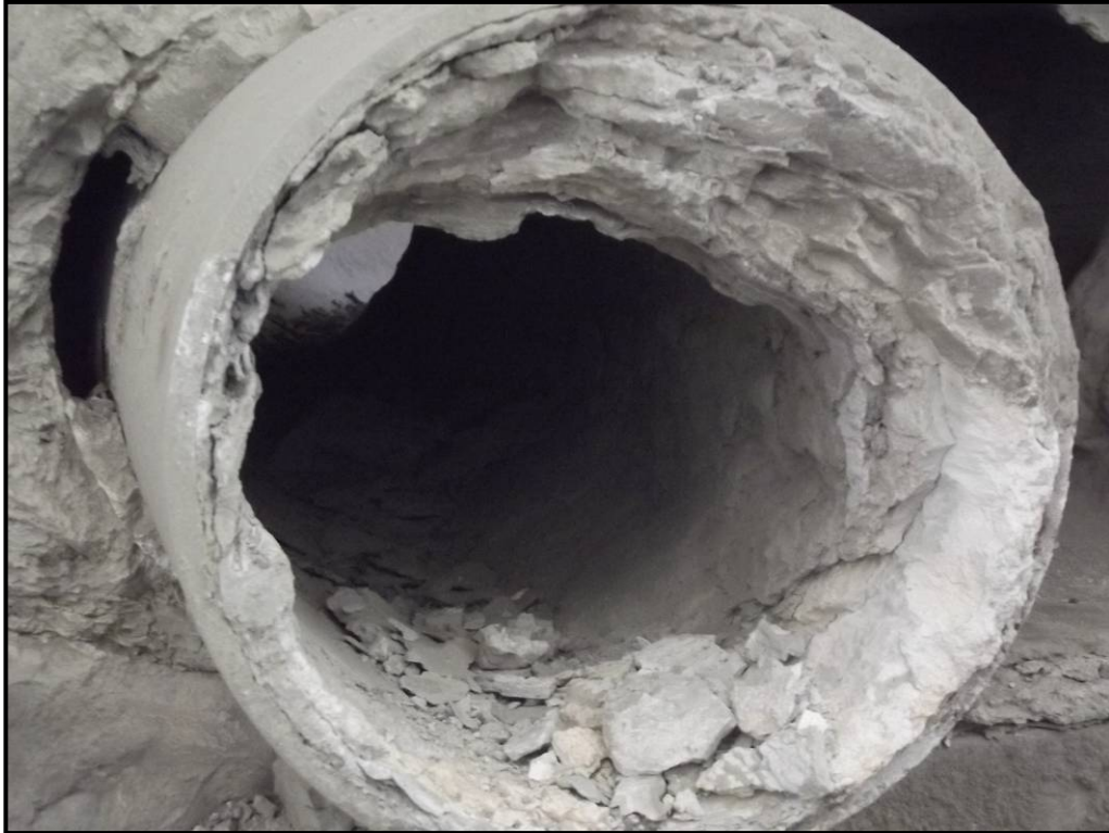
Photo 5 – Scale built up in pipes coming from the mills (recovered from Silo 12).
