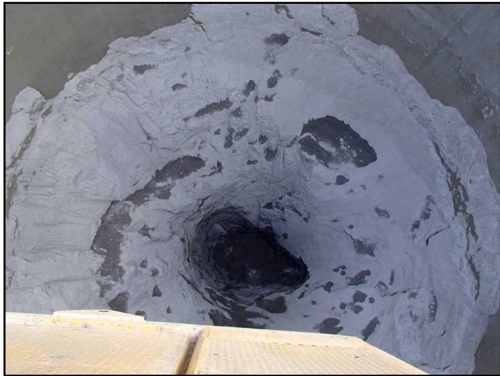
Photo14 – Bottom of rathole as of October 11, 2012, as the hardened material was removed.
