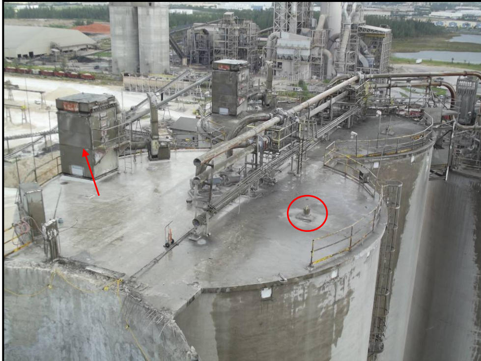
Photo 3 – Roof of Silo 11 showing dust collector position (arrow) and fan on the west side (left) and the feed pipe rack with F6 piping being the uppermost. The measuring port (right) is circled. Note all piping leading to Silo 12 (lower left) was removed during the recovery.
