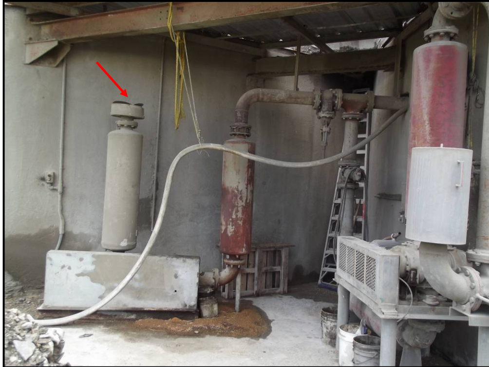
Photo 11 - Intake ambient air supply for the silo hopper air blaster. Cap (arrow) on intake filter was not attached.
