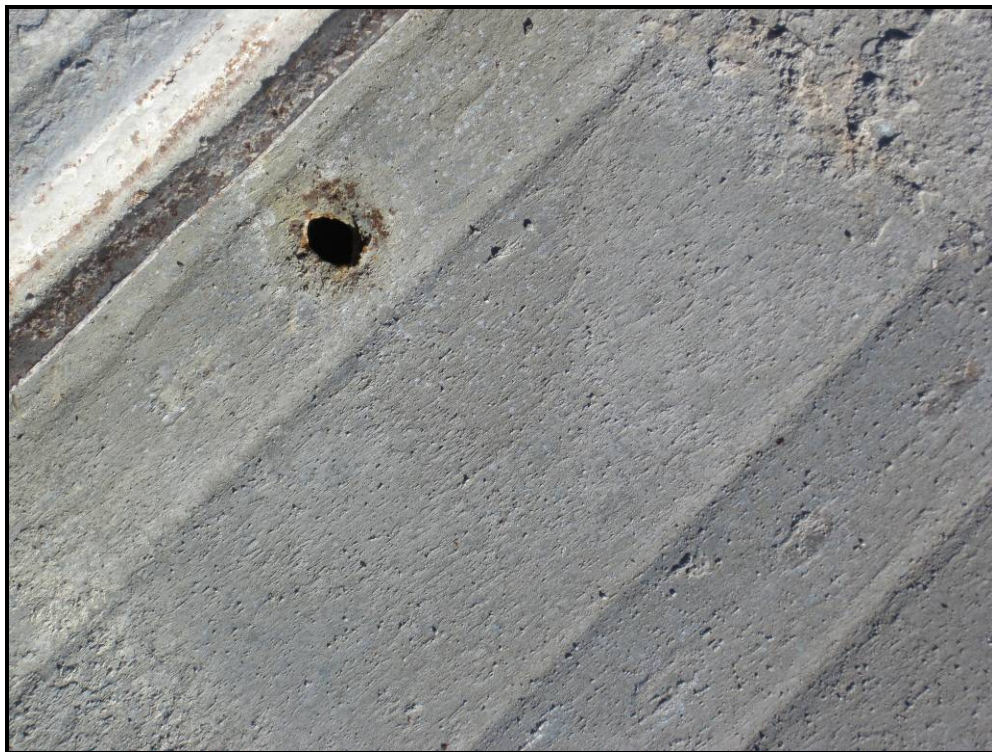
Photo 32 – Example of a decking failure around the weld. The decking was significantly corroded around the weld suggesting the failure had occurred prior to the day of the collapse. The decking metal will fail first when the weld is larger and stronger than the decking.
