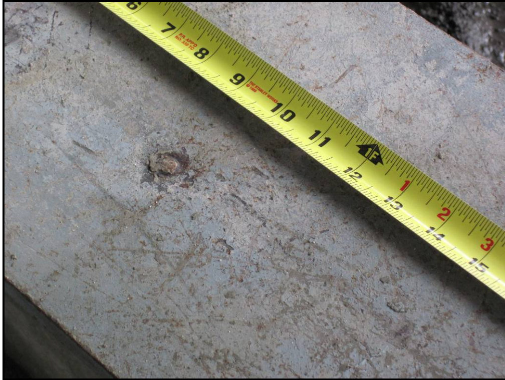
Photo 35 – Puddle weld with rubbed smooth failure surface on the top flange of Beam 5.
