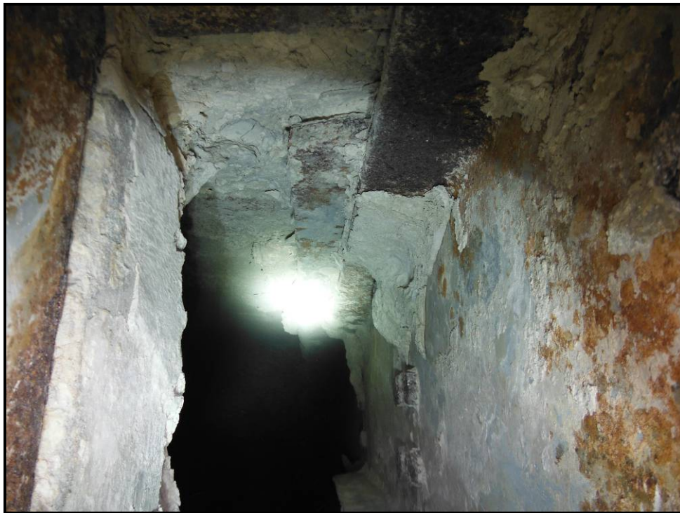
Photo 42 – View in East 3 pocket of Silo 11. Beam 3 is rotated south and slightly separated from the underside of the roof slab.
