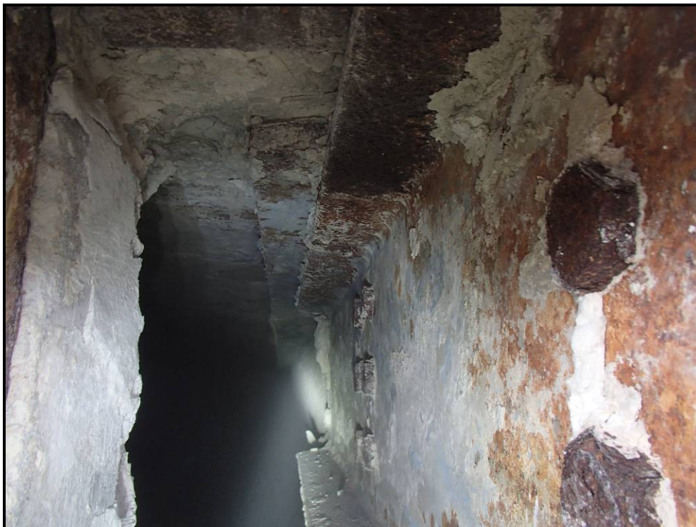
Photo 44 – Looking in East 4 pocket of Silo 11. Beam 4 is rotated to the left out beyond the end channel. A small gap existed between the top flange and the underside of the roof slab.
