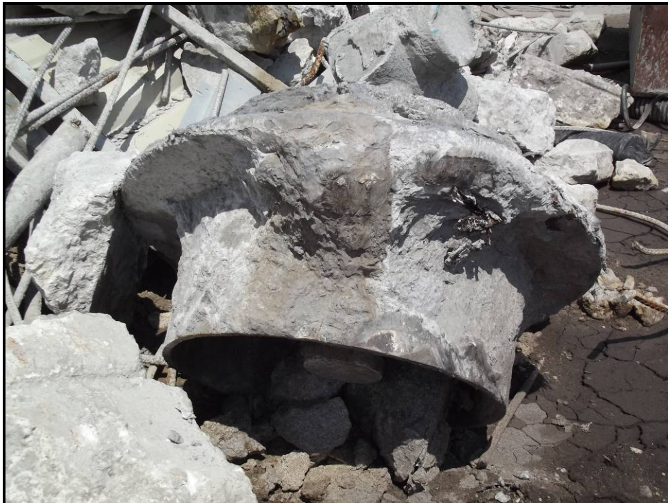
Photo 10 – An 18 inch radio transmitter level indicator from the roof of Silo 12. The top flange of Beam 3 was likely cut when this equipment was installed circa 2004.
