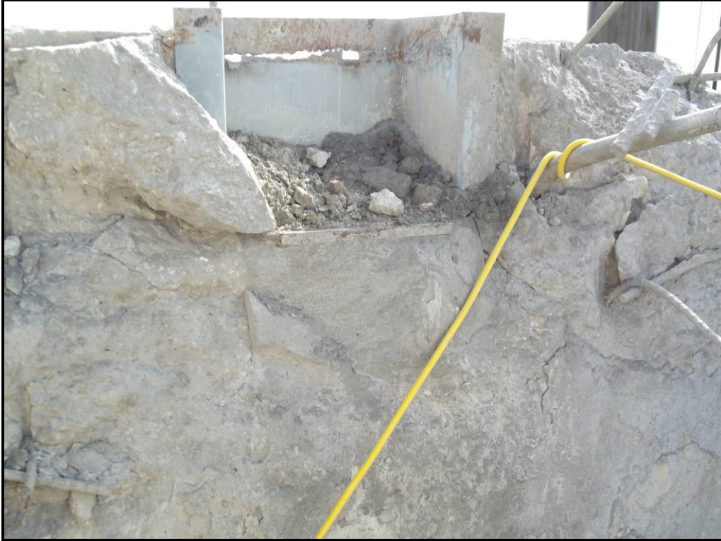
Photo 23 – Silo 12 East 6 pocket intact and no delamination detected in 10 inch-thick grout layer.
