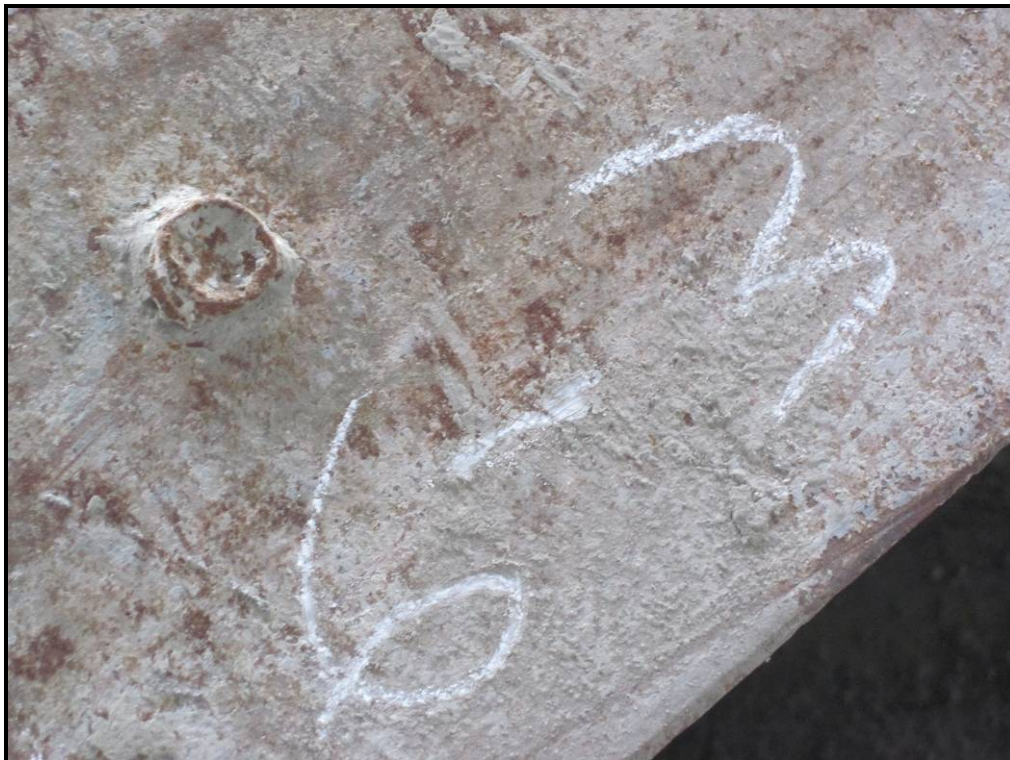
Photo 34 – Puddle weld failure on Beam 6 with a dished top surface. Weld was corroded, indicating that it had likely failed long before the day of the collapse.
