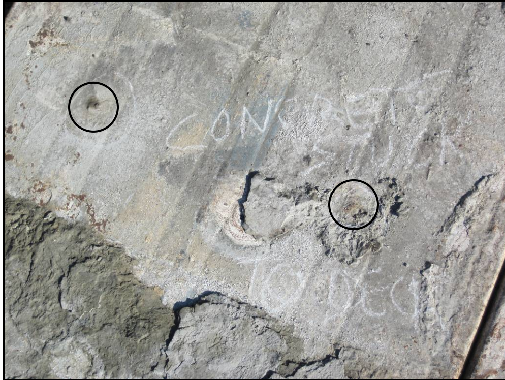
Photo 31 – Example of two puddle welds (circled) on the underside of the deck. The old residual hardened concrete next to the right weld indicates the weld had failed well before the collapse.
