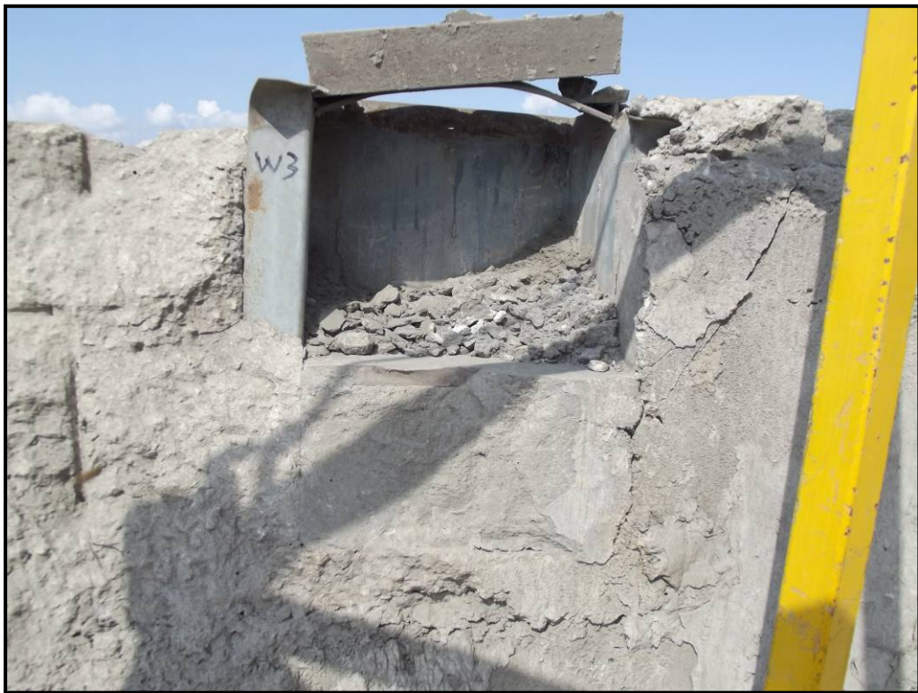
Photo 24 – Silo 12 West 3 pocket hidden delamination detected in 8.5 inch-thick grout layer.
