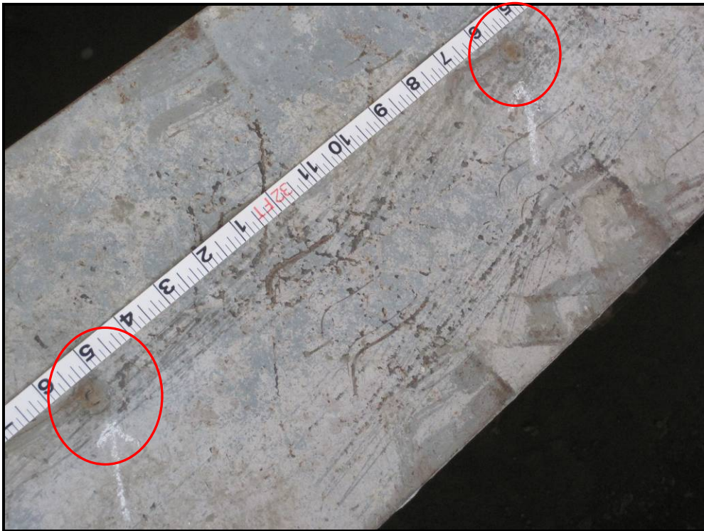
Photo 30 - Two faint markings where puddle welds did not adequately bond to the top flange of Beam 2 approximately 32 feet from the west end of the beam.
