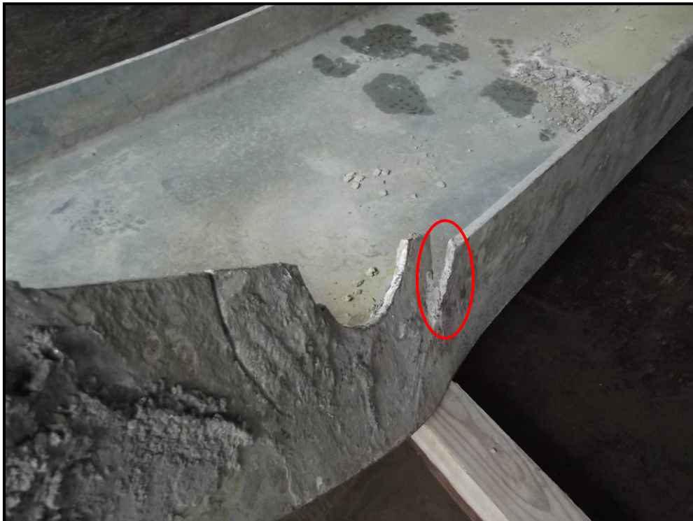
Photo 28 – Cut top flange of roof Beam 3 of Silo 12. Hardened concrete on flange and in the (circled) cut line indicate the beam had been buckled for some time prior to the day of collapse. Cut was likely made when the radio transmitter level indicator was installed circa 2004.
