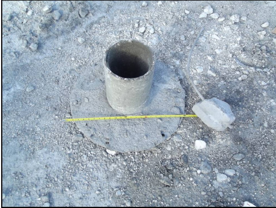
Photo 9 – Measuring port from Silo 12. Inside diameter measured 7-3/4 inches.
