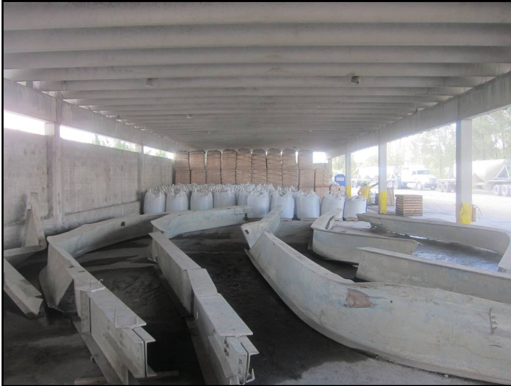
Photo 29 – Layout of Silo 12 roof beams. Beam 1 (only partly visible) is against left wall. Left to right is Beam 2 (2 sections), 4 (3 sections), 3 (2 sections), 5 (2 sections), and 6 (intact).
