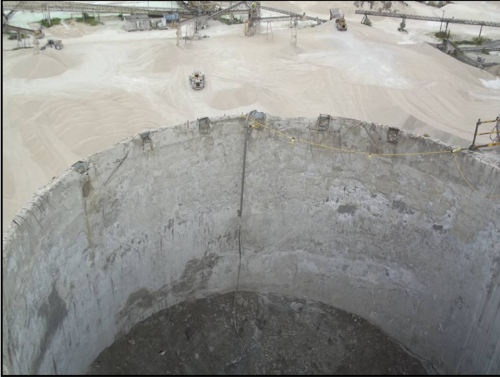
Photo 17 – Overview of the six west side beam pockets on Silo 12. Pocket W1 is on the left of the photo and Pocket W6 is on the right.
