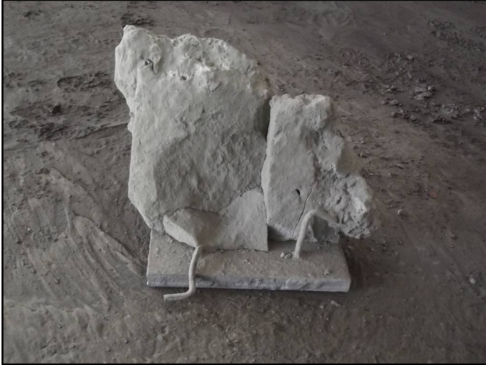
Photo 27 – Chunk of grout and bearing plate that sheared off. This plate was from either East 3, East 4, or East 5 pocket.
