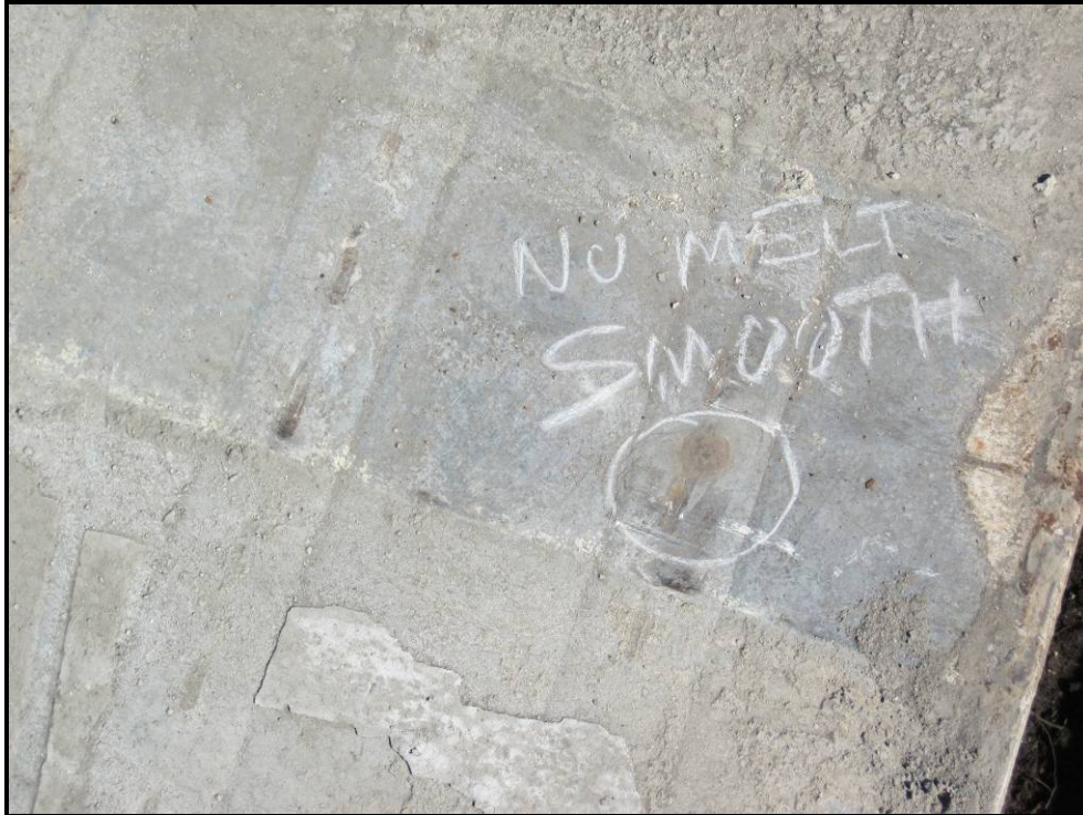
Photo 33 – Location where puddle weld did not penetrate the bottom plate of the roof deck.
