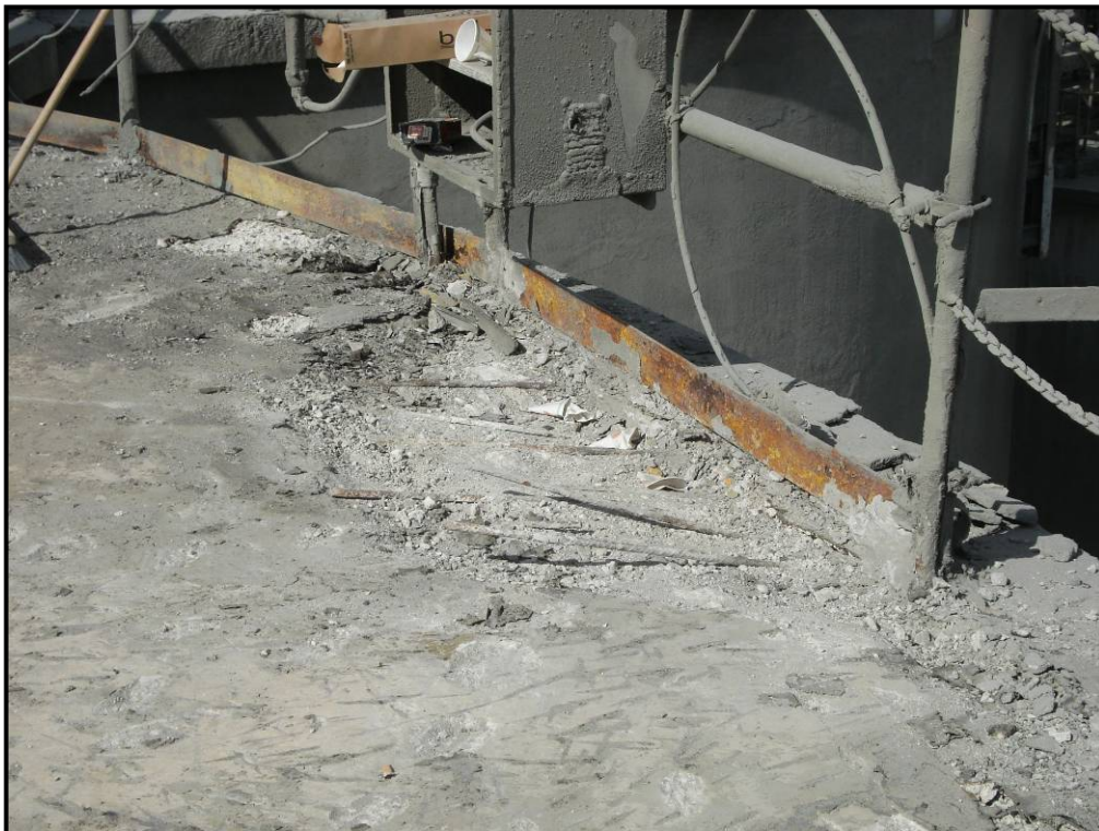
Photo 4 – Damage to Silo 11 roof when it was over pressured in 2011. The roof bulged and the bent over vertical reinforcing bars popped out of the slab at the perimeter when the roof relaxed.
