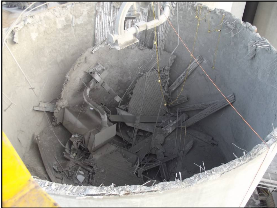
Photo 16 – Looking toward north wall. Photo taken 1 day after Silo 12 collapse. Large slab section still attached to the dust collector would have spanned from Beam 3 to the north wall.
