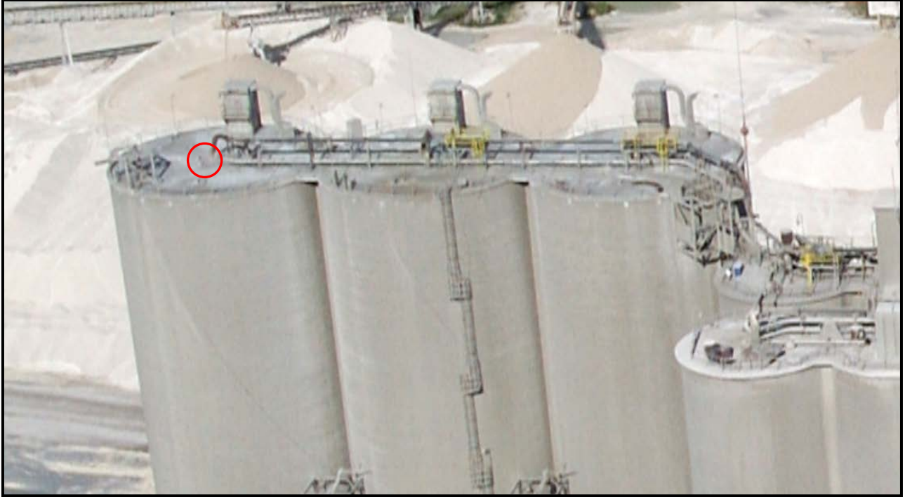
Photo 15 – Overview taken in 2004 looking at the east side of Silo 12 (left), 11, and 10 roofs. Circled area shows two ports on Silo 12. The upper left port was an observation port as per the original drawings and the lower right port was for a radio transmitter level indicator added (circa 2004). Note this photo was taken prior to the addition of F6 mill piping.
