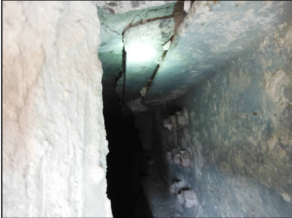
Photo 41 – View in East 2 pocket of Silo 11. Beam 2 has a rotated top flange that is separated from the underside of the roof decking by approximately 1 inch.
