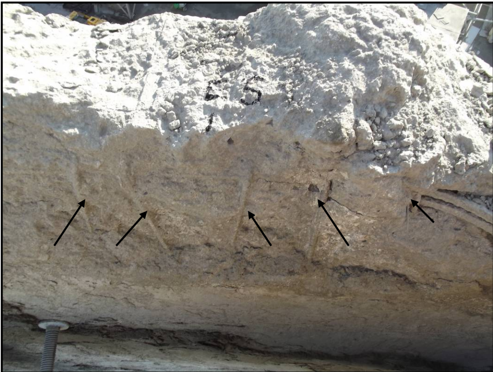
Photo 22 – Silo 12 East 5 pocket completely torn from silo wall above the location of the shear stirrups (arrows)
