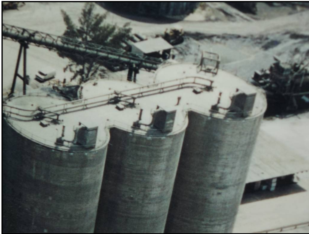
Photo 2 – Silo 10 (left), 11, and 12 (circa 1996). This was prior to the MCC and F6 mill piping being added.
