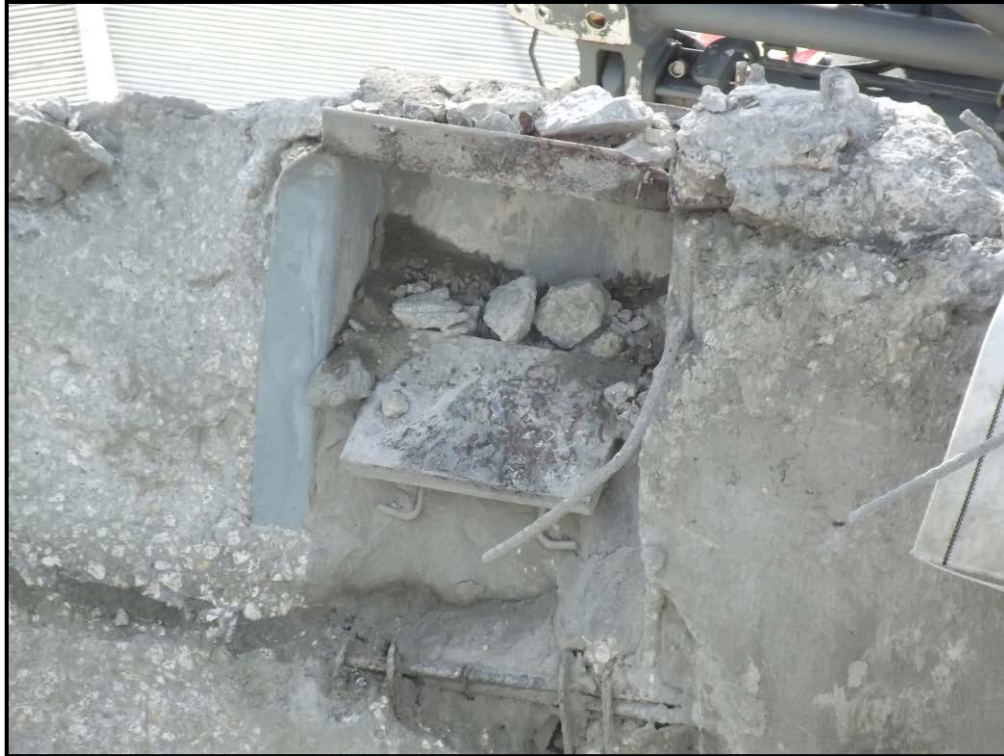
Photo 19 – At East 2 pocket of Silo 12, the grout sheared below the front half of the bearing plate and it tilted downward. Note honeycombed concrete void below the exposed shear stirrups.
