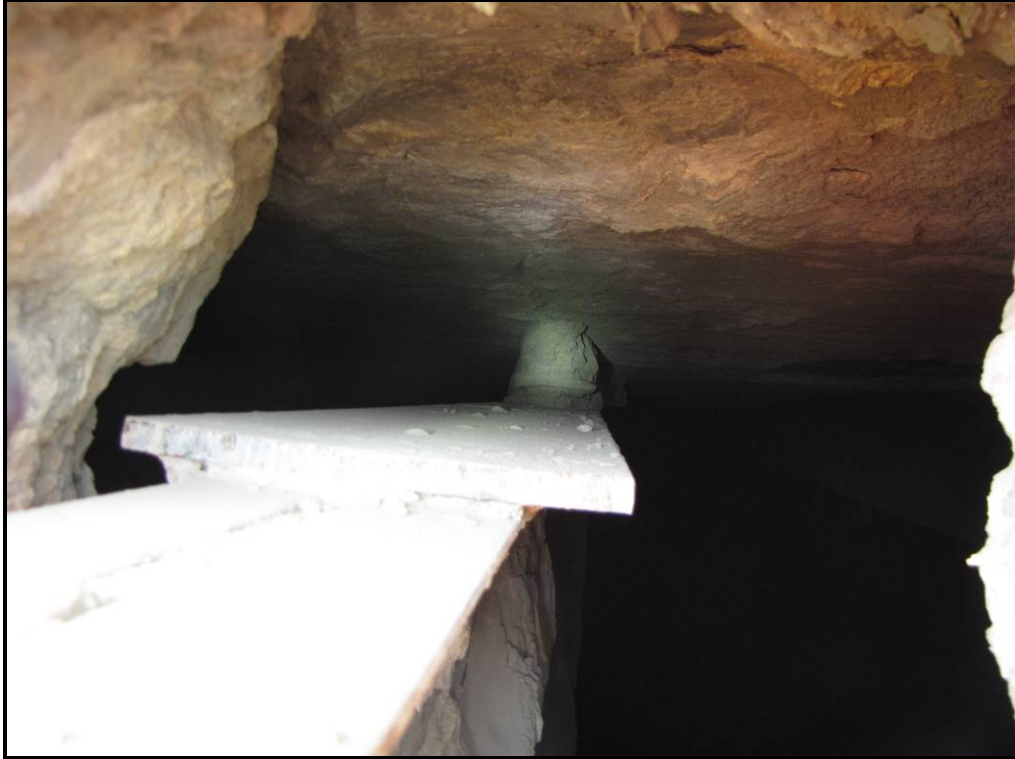
Photo 39 - View looking in East 3 pocket of Silo 10 at separation between Beam 3 and the underside of the roof slab.
