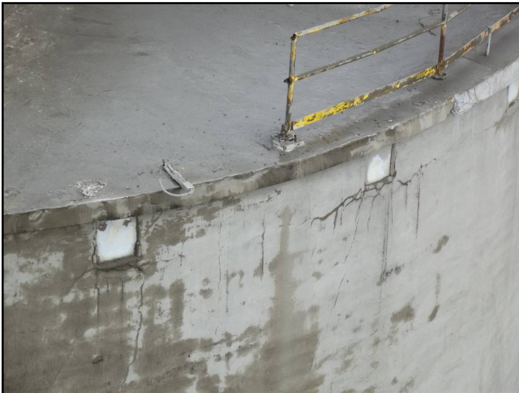
Photo 26 - Cracking at the beam pockets on the east side of Silo 11. This cracking was typical on all three silos.
