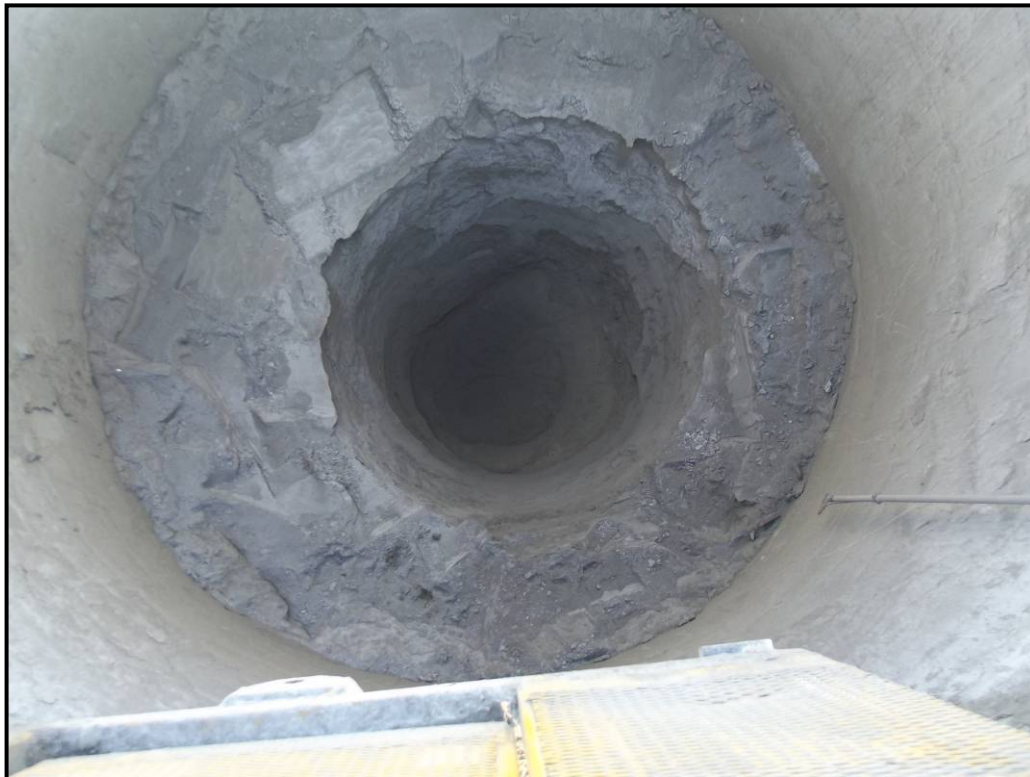
Photo 12 – Stable rathole revealed as Silo 12 was drawn down. Picture taken on September 11, 2012.
