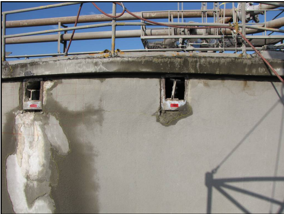
Photo 38 – Silo 10 beam pockets E3 (left) and E4 (right). Neither Beam 3 nor 4 was in contact with the roof. Beam 4 is also significantly rotated.
