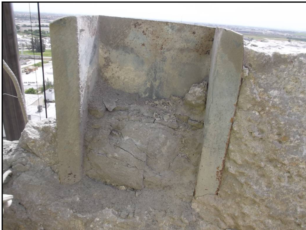
Photo 20 – Grout delaminated and sheared off at Silo 12 East 3 pocket. Multiple cracks present in 11 inch-thick grout layer.
