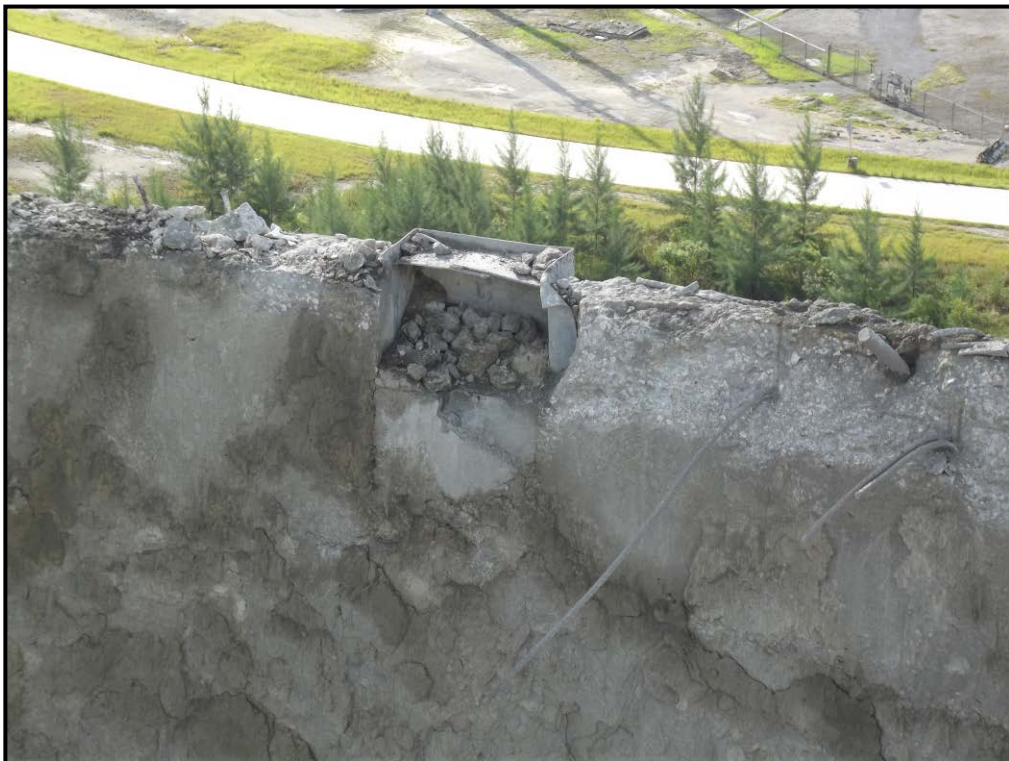
Photo 18 – East 1 pocket of Silo 12 was intact, but near surface delamination detected in 10 inch-thick grout layer.
