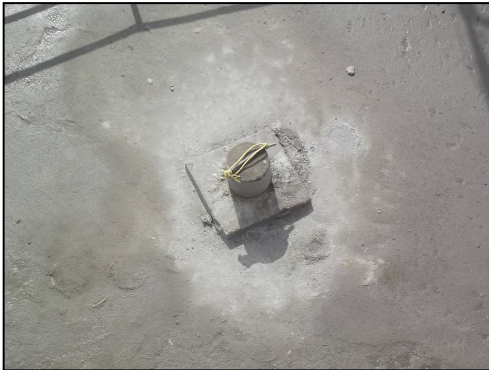
Photo 8 – Typical measuring cap for Silos 10, 11, and 12. Cap weighed 60 pounds and also acted as a pressure relief device.
