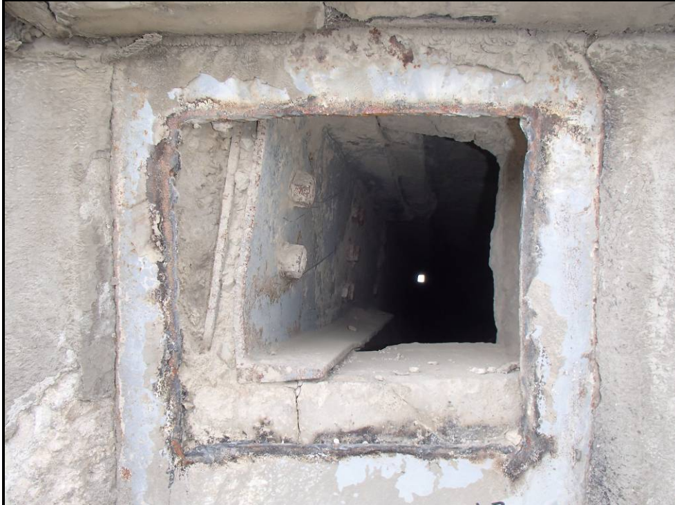
Photo 43 – Rotation of the end channels and roof Beam 3 along with cracking of the grout pad at the West 3 pocket of Silo 11
