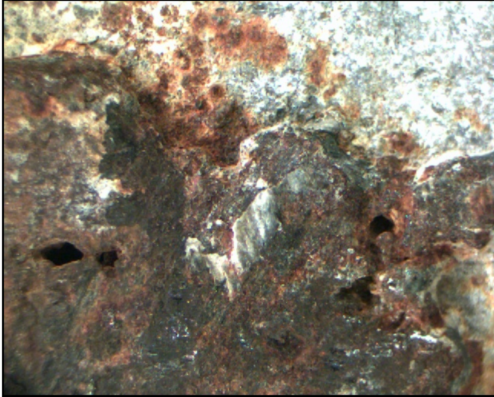
Photo 37 – Porosity and old corrosion on the failure surface of puddle weld M1. The weld was still attached to the underside of the metal decking.
