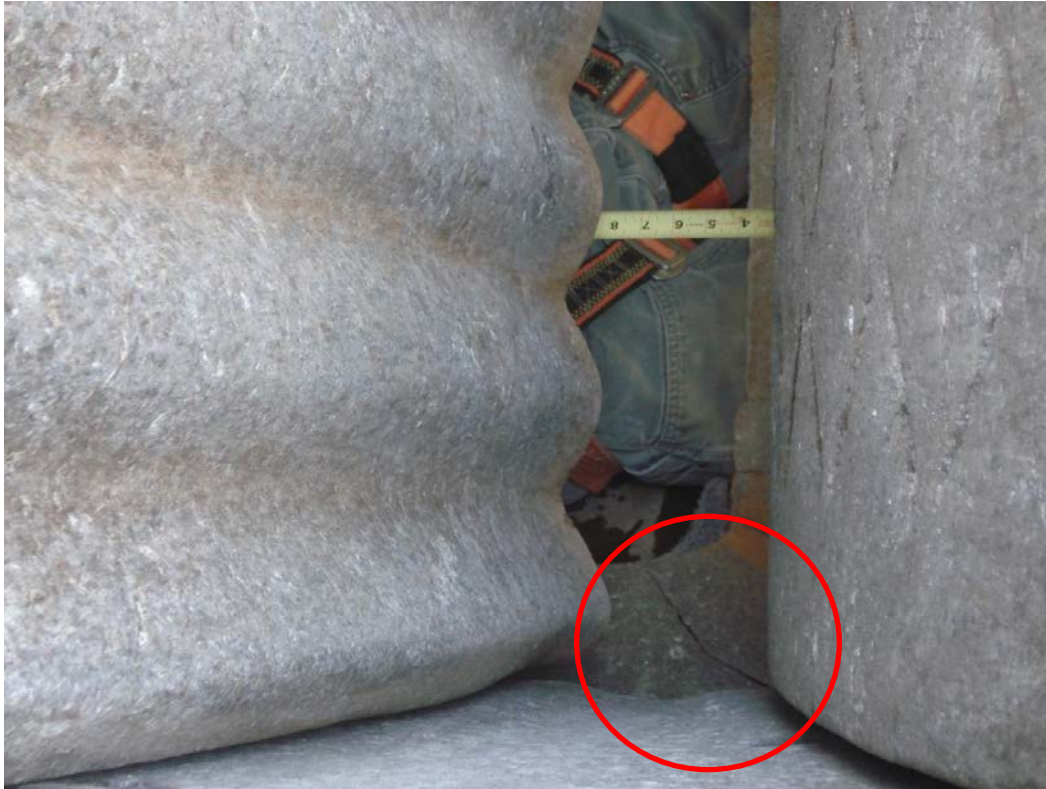
Figure 2 - A very large crack (as shown) in the steel frame of the throat of the jaw crusher. (Note: An accident investigator appears in the photo.)
