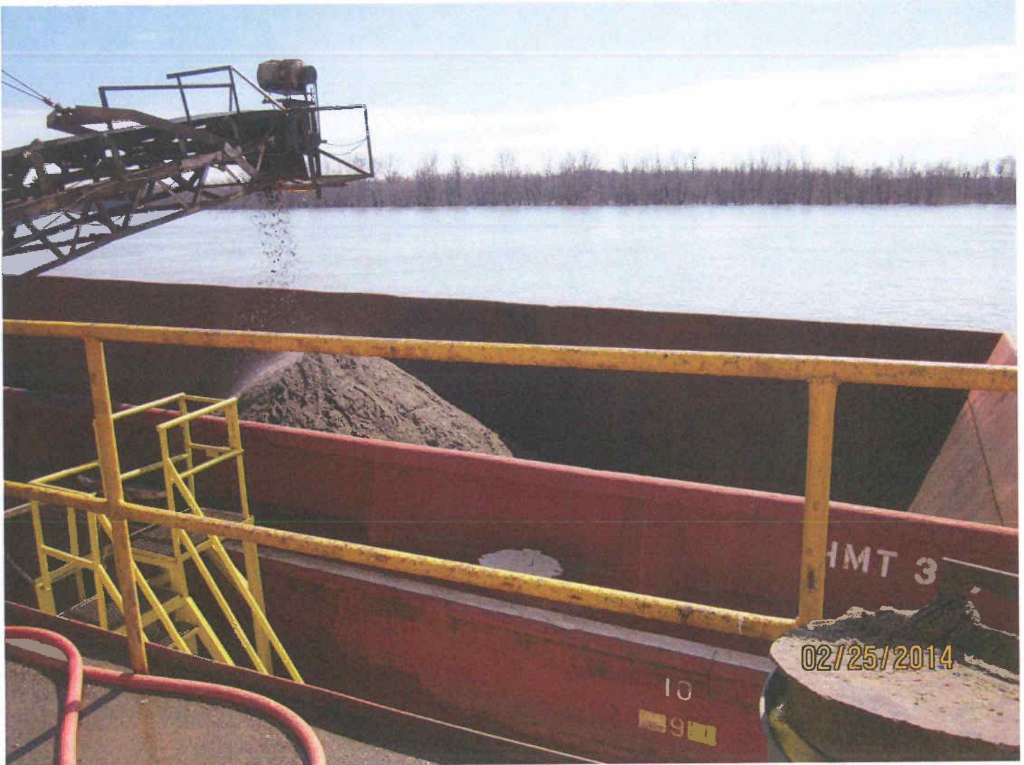
View of barge being loaded from the control room landing of Dredge IV. This is what the operator sees with the control room door open. The stairway shown on lower left is how the deckhands access the barges.
