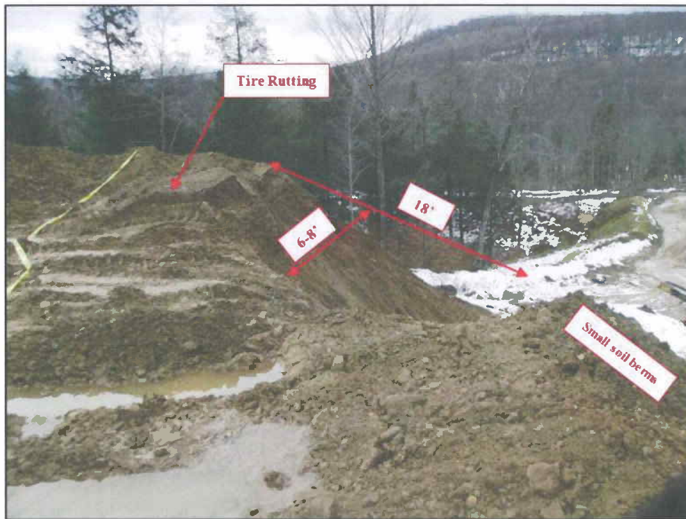
Figure 10 - Localized slope failure which occurred beneath the rear tires of the haul truck. Deep tire ruts show minimal strength of wet, soft, cohesive material comprising the dump surface and soil berms.
