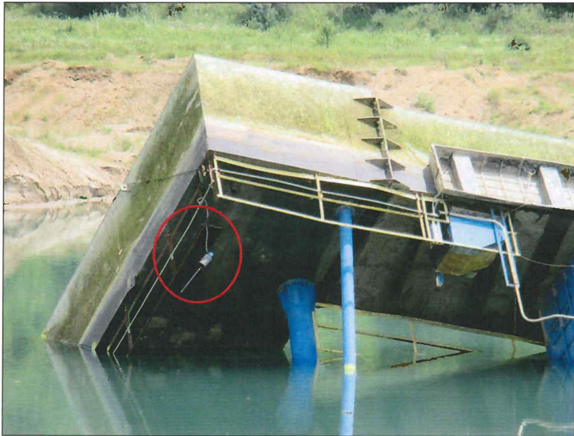
Figure 4 - Dredge in water. Note missing hatch cover and hanging overload sensor.
