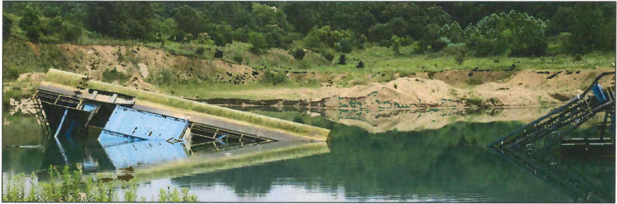
Figure 3 - Dredge in the water at the beginning of the investigation.
