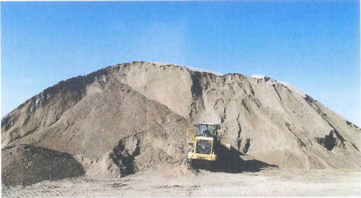
Figure 2 - Stockpile and Slide
