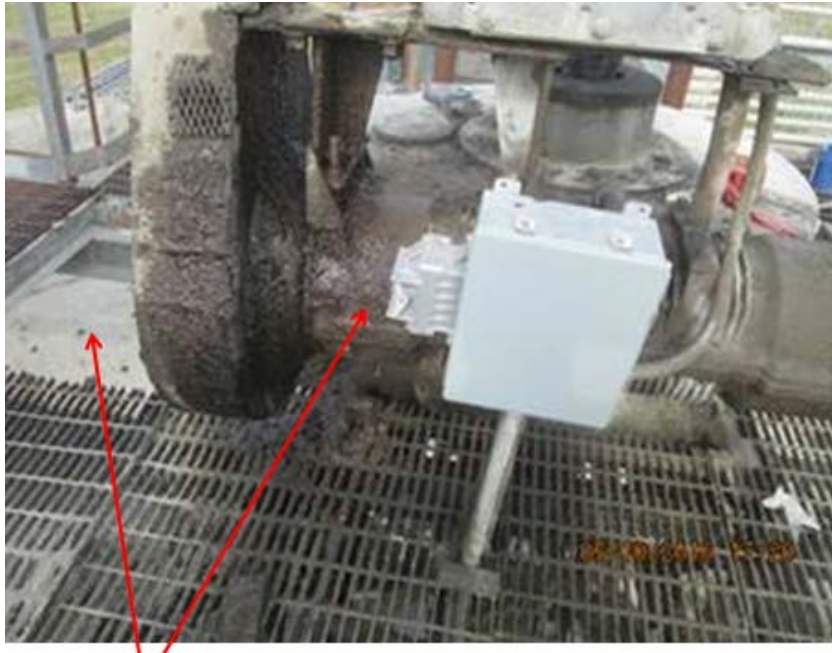
Arrows indicate missing grating and control switch to be used to move rakes
