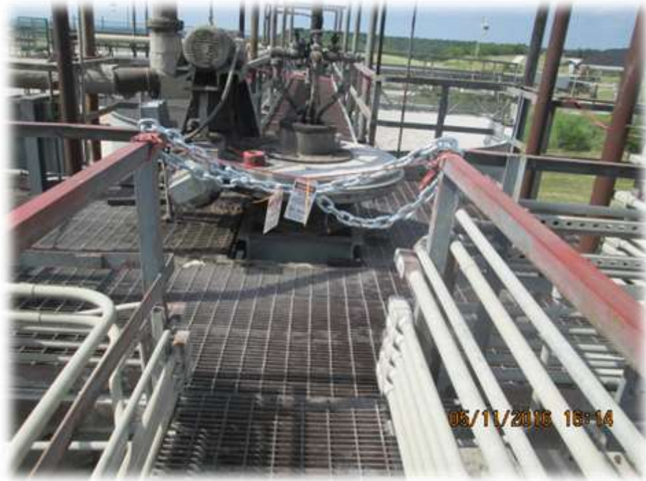
Attachment #2 (Entrance to work site)
