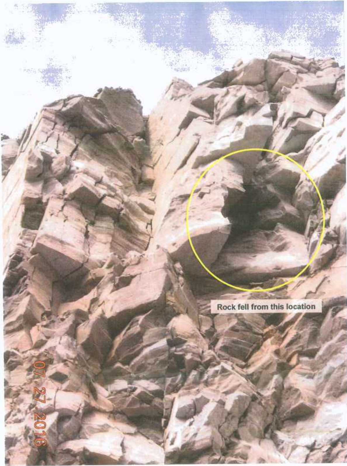
Photo 2 Close-up View of Rockfall Origination and Highwall Face
