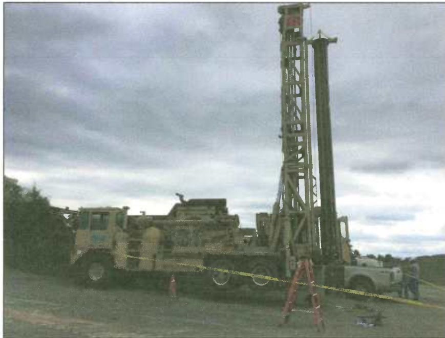
Figure 2 - The Ingersoll-Rand/Atlas Copco Model T4BH Drill Rig (overview)
