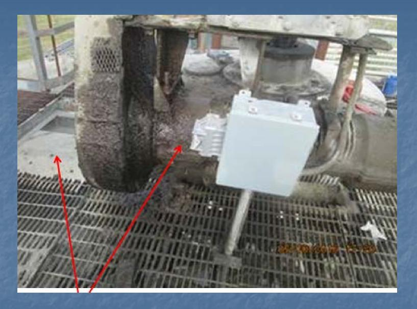
Arrows indicate missing grating and control switch to be used to move rakes
