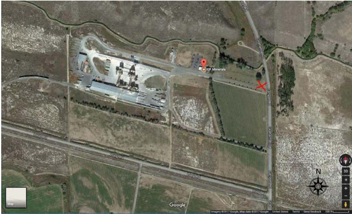
Figure 1 – Overhead view of the EP Minerals, Celatom Plant. The red “X” was used to show the approximate location of the accident.
