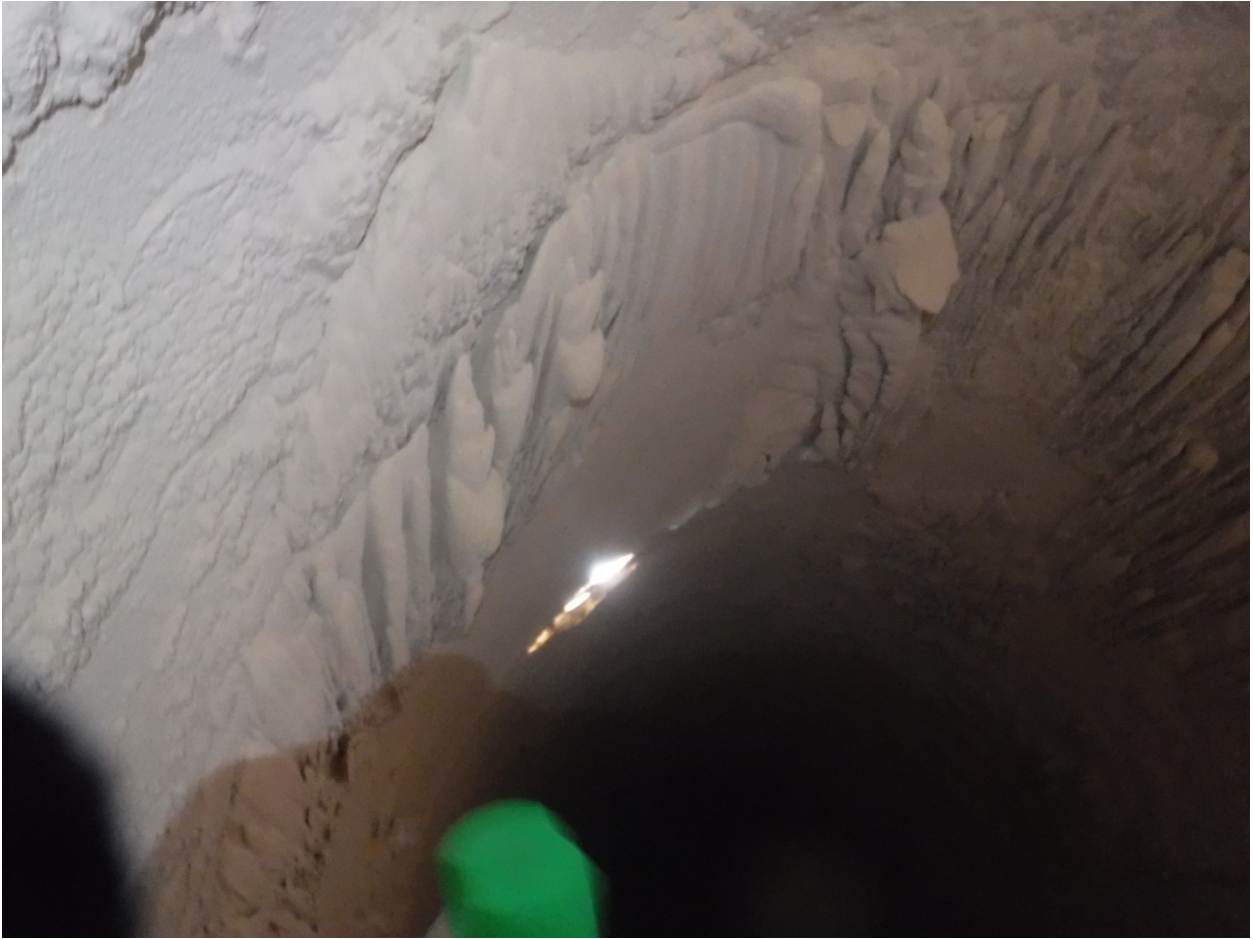
Photo 1 – Material caked on duct walls
