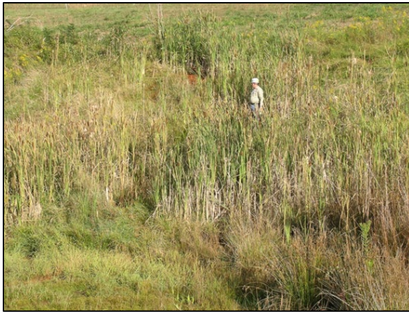
Photo 21. Cattails and lush vegetation are potential signs of seepage.
