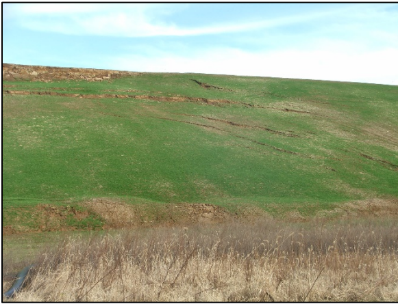
Photo 23. Cracks on embankment slope.
