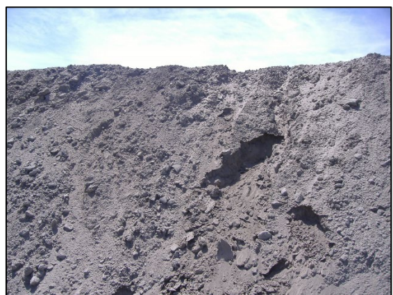
Photo 10. Poorly compacted tailings embankment raise.
