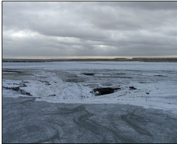
Photo 13. Sinkhole in pool area.
