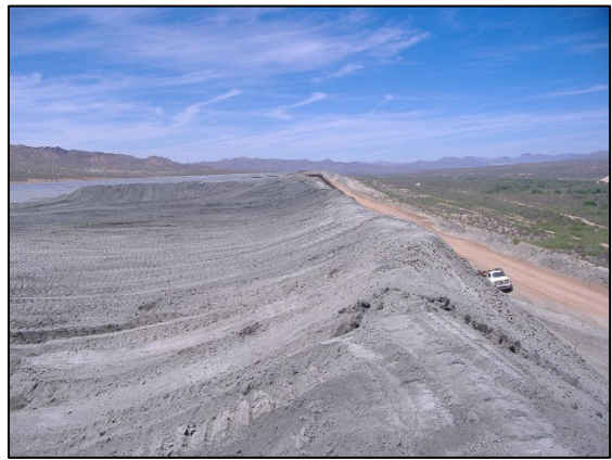
Photo 8. Compaction of tailings dam raise.
