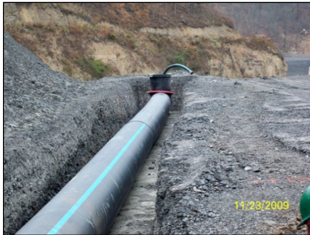
Photo 14. Principal spillway installation in trench.
