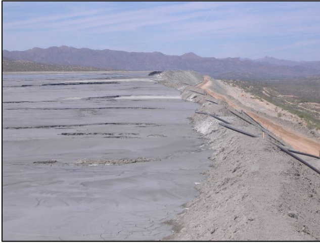
Photo 12. Discharge lines for placement of tailings along the upstream slope.
