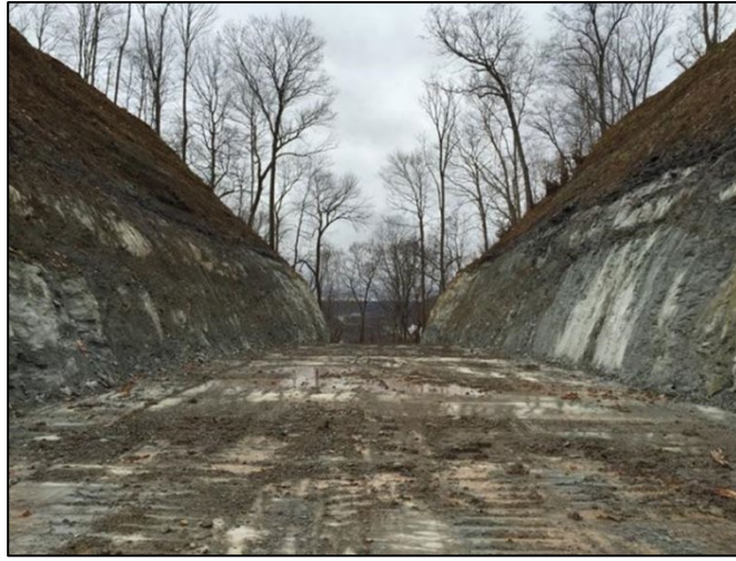
Photo 19. Open-channel spillway excavated in rock.
