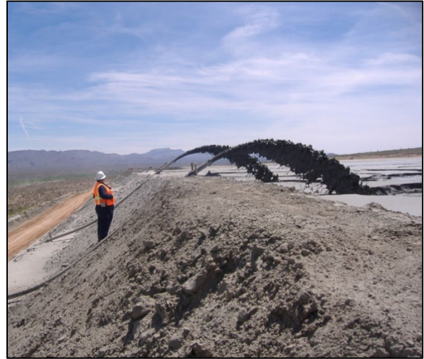
Photo 4. Delivery of waste to a metal and nonmetal tailings dam.
