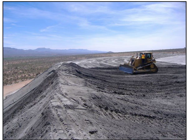
Photo 2. Construction of a metal and nonmetal tailings dam embankment.
