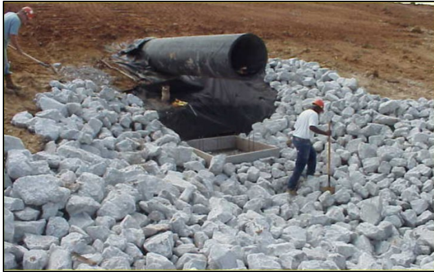
Photo 25. Construction of erosion protection at pipe outlet.
